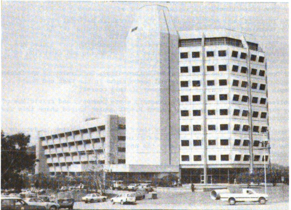
Government buildings, Waigani. The one on the right is known locally as the 'Pineapple Building'
