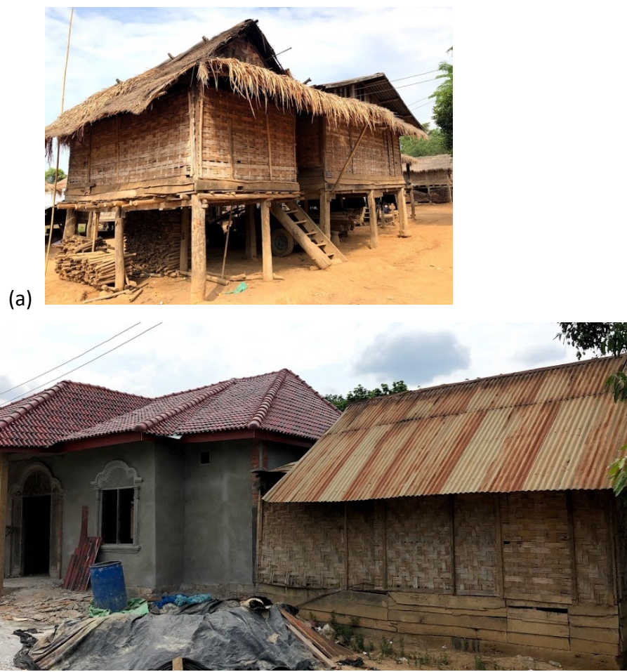
Figure 2.2: Picture (a) the most common traditional housing (bamboo wall with a grass roof) in upland communities; (b) new concrete house (next to the old house) after the arrival of cash crop production (bananas). Namox District, Oudomxay Province, Northern Laos
