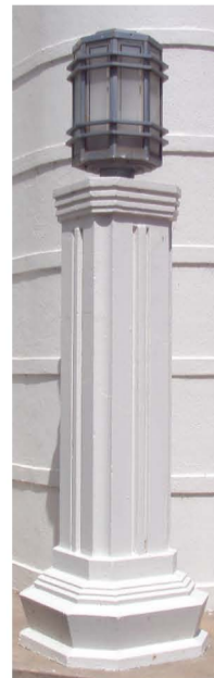
Decorative lighting features
