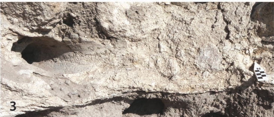
FIG. 12 Examples of Middle Byzantine defensive wall construction using deadmen when needed: (1) Trench SMT 15, note only one or two deadmen used above Late Iron Age architecture mudbrick wall on right; (2) Trench SMT 4, note “box” used to support wall, outlines of which are visible above the number in lower right corner; (3) close-up of hole showing grain pattern of deadmen lying beneath defensive wall. (Photos courtesy of the Çadır Höyük Excavation.)
