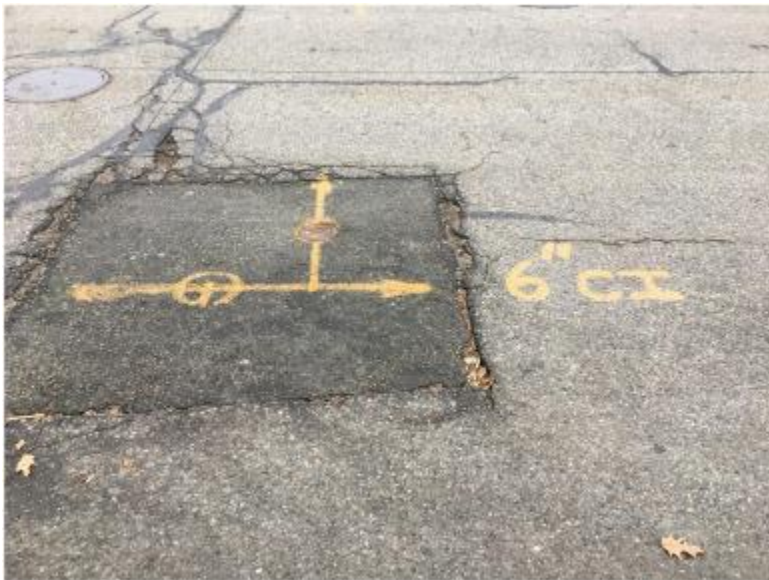
Fig. 5.3. Example of a spray painted marking on a road by utility company.
