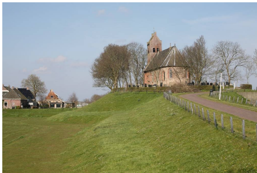
Figure 7. Hegebeintum (Frisia), the 12th-century church sits on top of an 8.8 m high mound, called a “terp” (photo: Regnerus Steensma archive).
