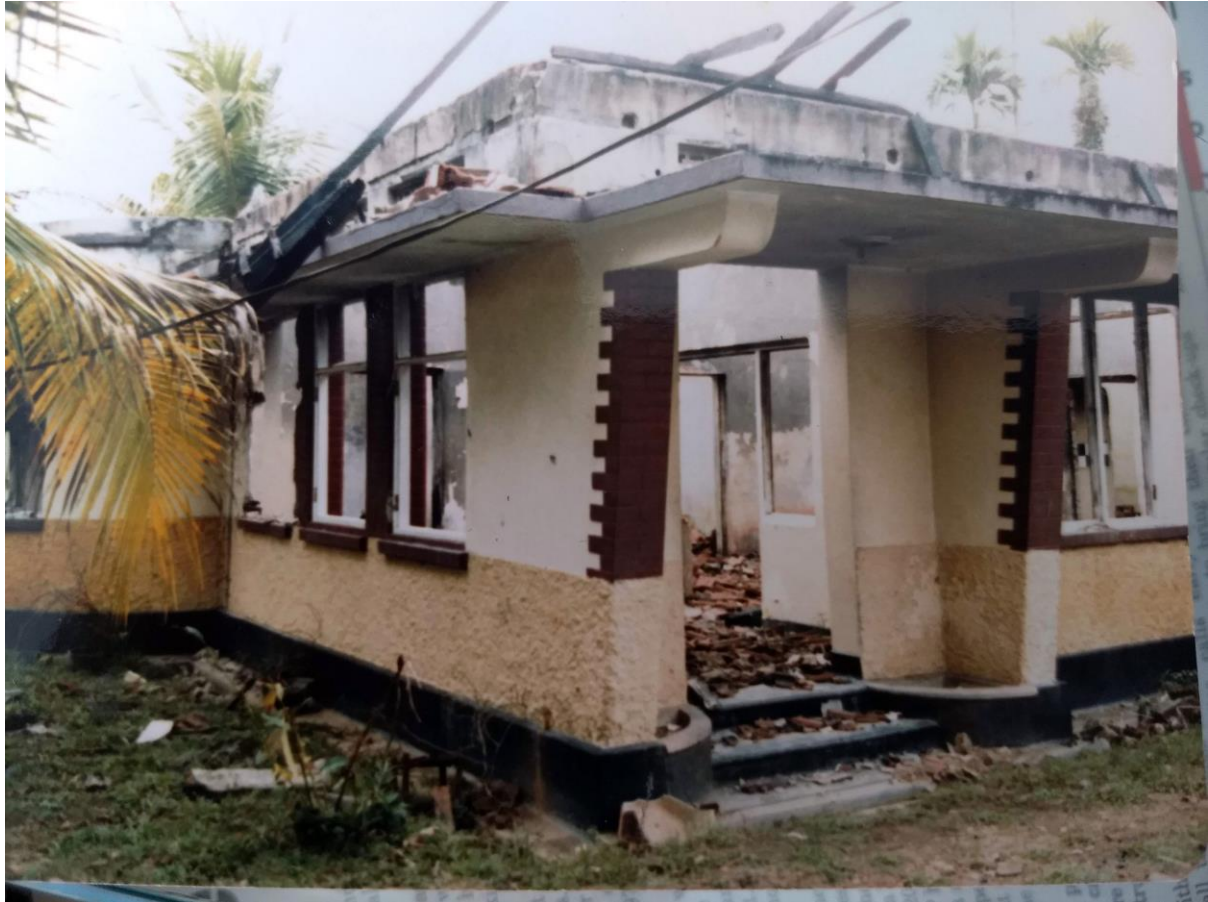
MN's destroyed house, Colombo, 1983.
