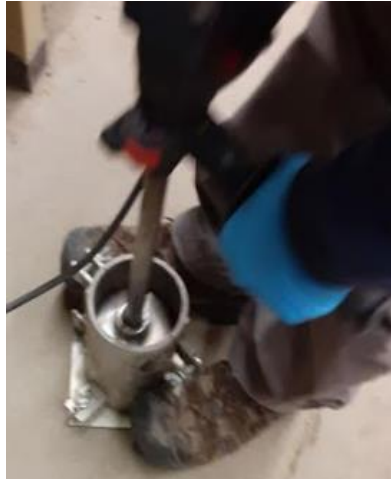
Figure 25. Compaction with Vibratory Compactor.
