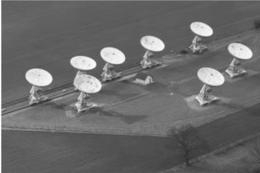
Figure 3.1: LA from the north-east. The correlator is in the central hut. The railway track, which runs diagonally across the photograph, is approximately east-west. Four antennas are moveable along the track. Ref: (Zwart et al., 2008).
