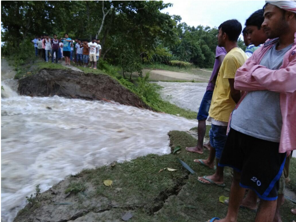
Fig. 2.2. Residents look on and take photographs as the breach expands and the inner grazing lands, and this side of the village, is rapidly flooded (source: Papu).
