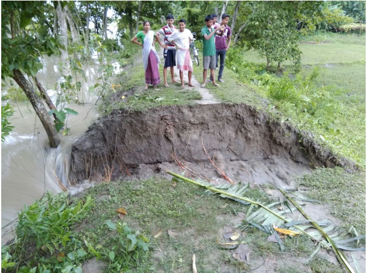
Fig. 2.1. A few moments after the top of the embankment caves in on itself (source: Papu).
