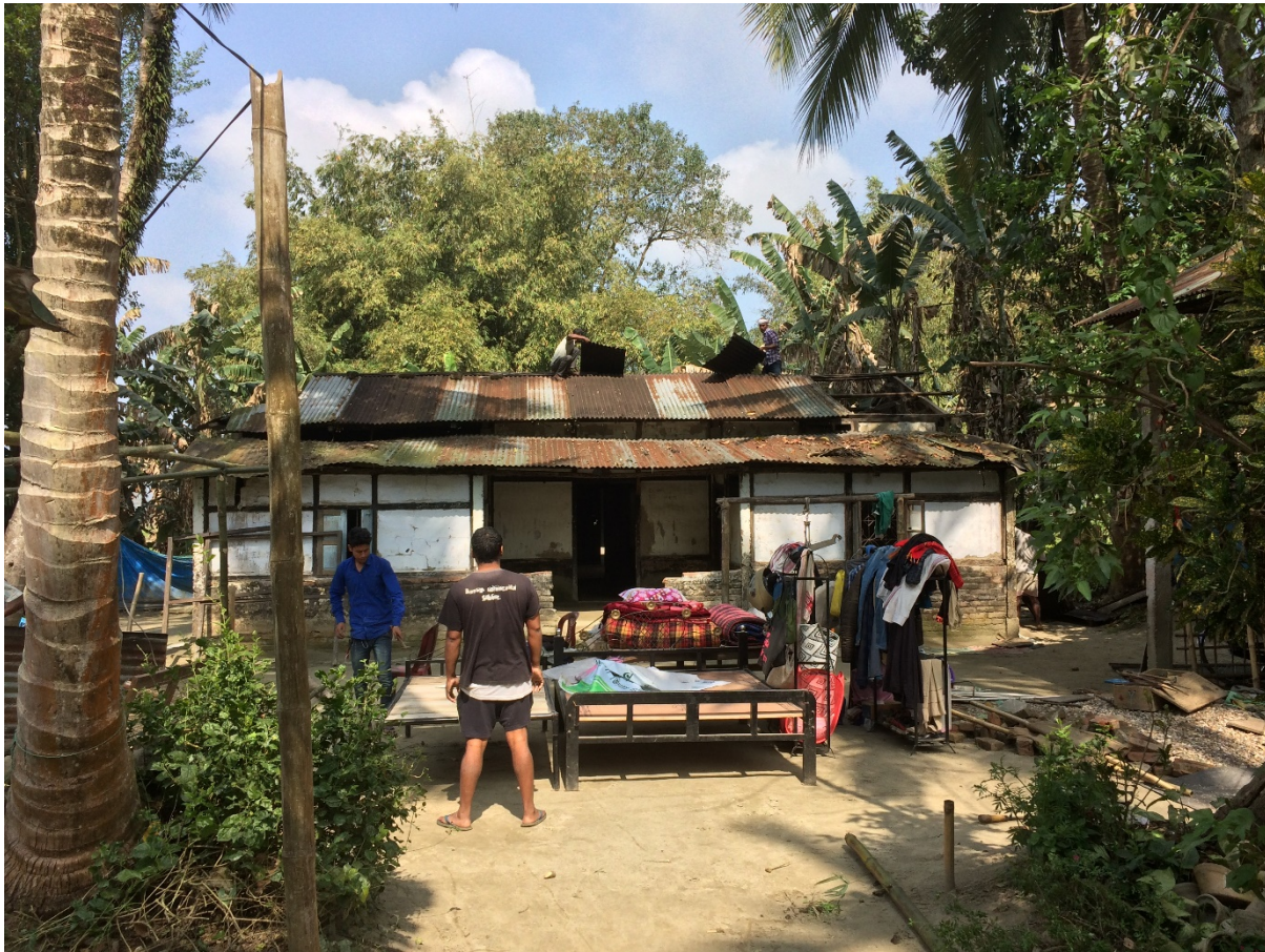
Fig. 3.1. Belongings outside old house, as labourers began the demolition.
