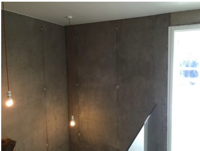
Figure 38: The H-cores in exposed concrete after the renovation
