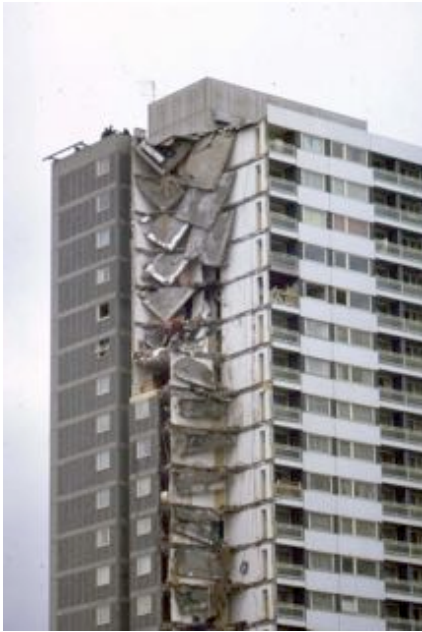
Figure 13: The collapse of Ronan Point. Image taken from Geograph.org.uk
