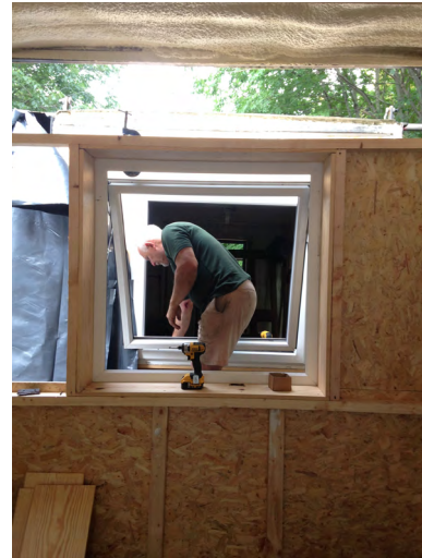
Figure 6.1.3 - UPVC window installation.
