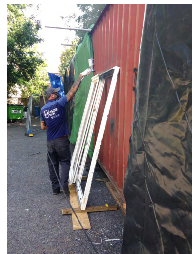
Figure 6.2.2 - L to R, Chipping the UPVC paint with a fingernail, spraying the UPVC with more resistant paint.
