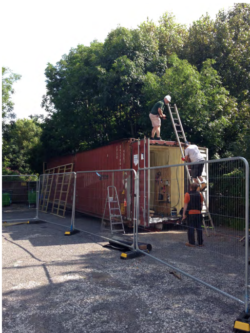
Figure 6.1.2 - Paid REACH labourers, the construction team.
