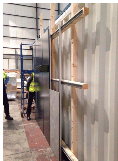
Figure 6.1.4 - Clip on facade system.
