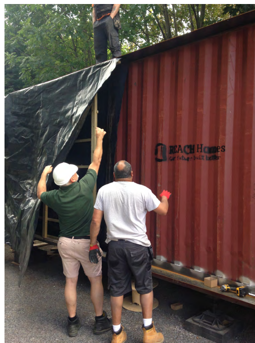
Figure 6.1.3 - Trying Billy's idea, lapping the membrane around the insulation frame.
