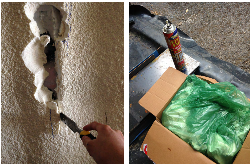
Figure 7.2.2 - Taking off the waste insulation and testing a new insulation block.
