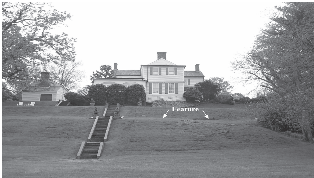
Figure 12. The rear of the Sentry Box showing the 1920s terracing. (Photo by Dovetail Cultural Resource Group, 2008.)
