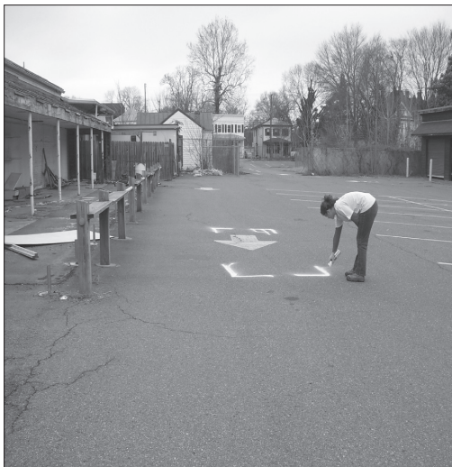
Figure 3. Marking the locations of backhoe trenches at the Fredericksburg Hardware Store site. Trench locations were based on archival research. (Photo by Dovetail Cultural Resource Group, 2007.)
