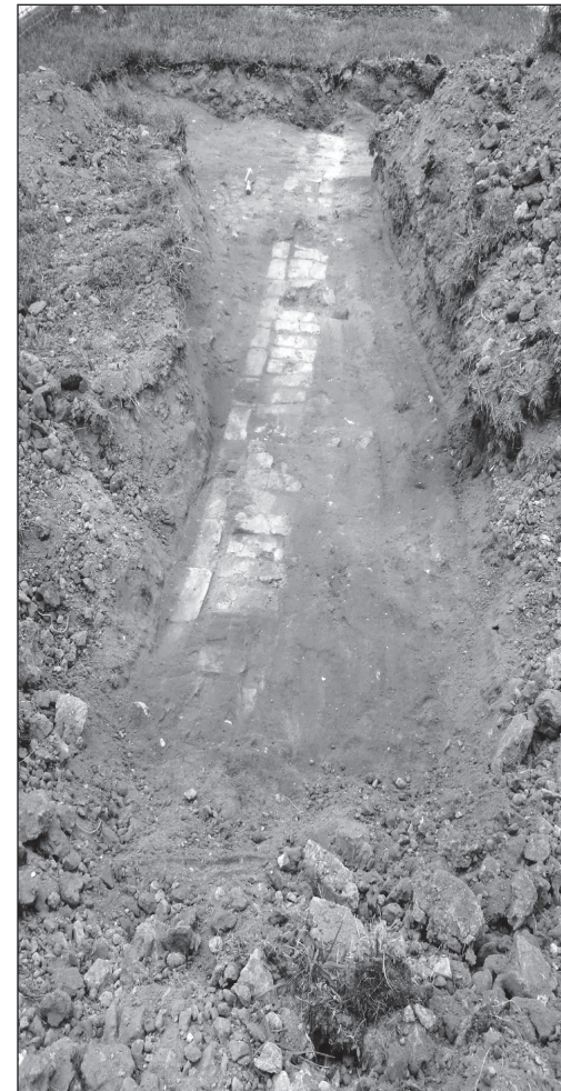
Figure 14. Foundation of a brick duplex at 717-719 Sophia Street in the Riverfront Park area, identified through backhoe trenching. (Photo by Dovetail Cultural Resource Group, 2013.)
