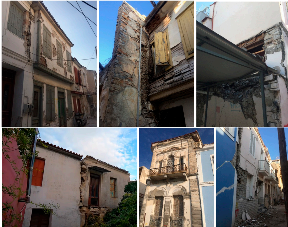
FIGURE 7 | Examples of pounding induced damage in timber-masonry structures [DG2-DG3] (Samos, Greece) Examples of pounding induced damage in timber-masonry structures [left picture from Mikres Diadromes Samou, 2020] [DG2-DG4] (all in Samos, Greece).
