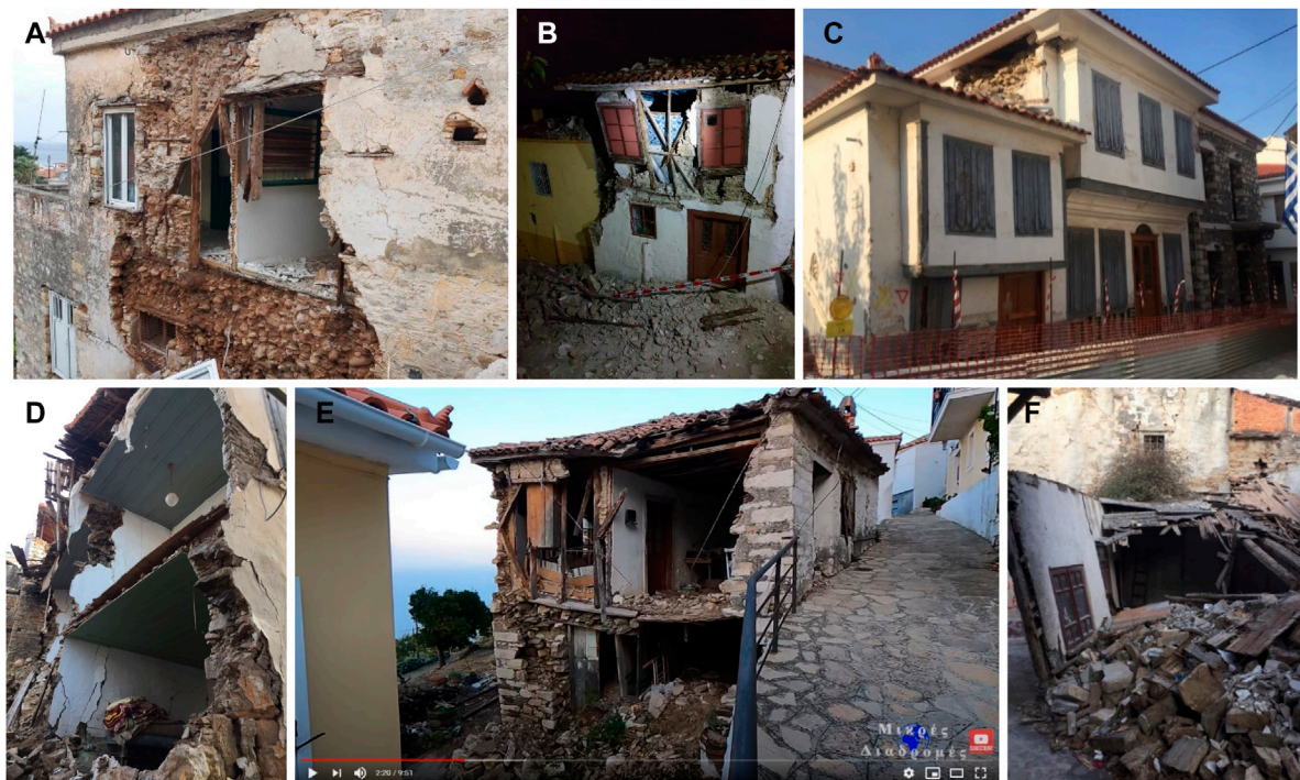
FIGURE 2 | Examples of timber-masonry structures which suffered from failure of masonry: (A–C) out of plane infill failure of masonry in the upper floors, (D,E) failure of masonry ground floor and timber frames above (F) total collapse induced by the failure of the masonry ground floor [( B,E ) from Mikres Diadromes Samou, 2020] [DG3-DG5] (all in Samos, Greece).
