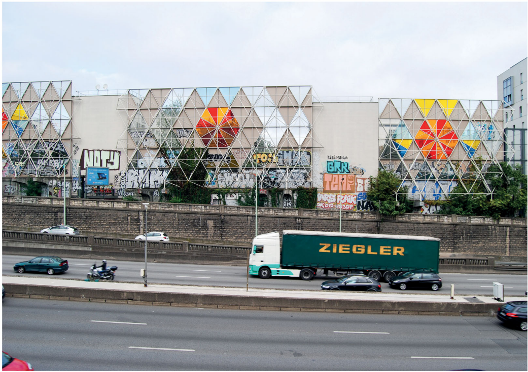
Figure 3. Sound walls 'Maryse Bastié', near Porte de Choisy, built in 1989 (2017–2022, Courtesy of the author).
