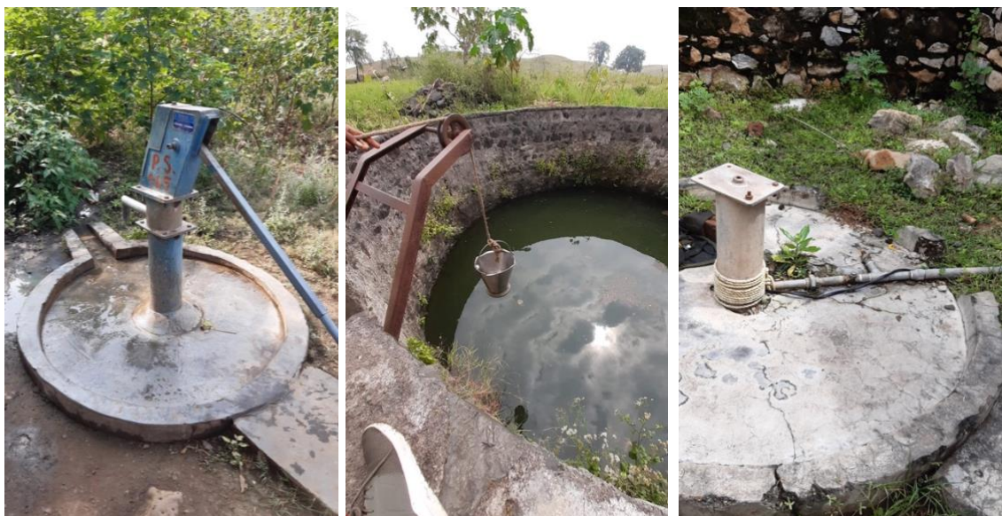
Image 5-5 Domestic water sources: Mechanical hand-pump (left). Unimproved open well (centre). Electrical borewell (right).
