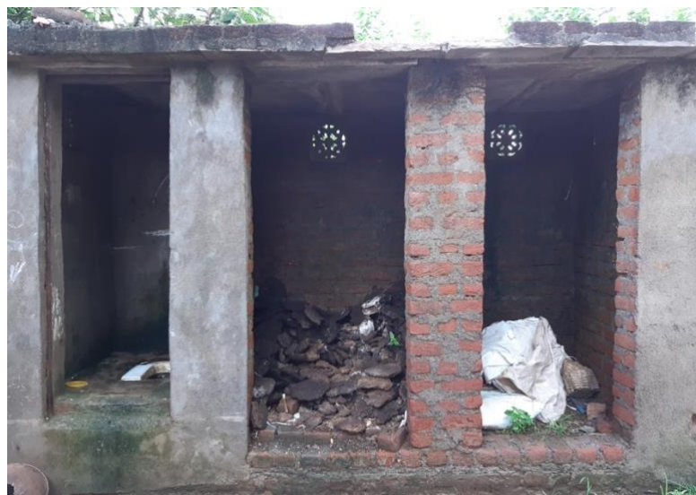
Image 5-6 Example of an unfinished latrine construction
