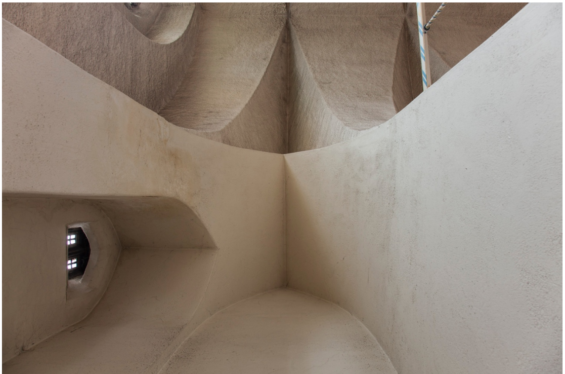
Fig. 39 Ceiling detail at St Thomas the Apostle Church (David et al. 2015:224)
