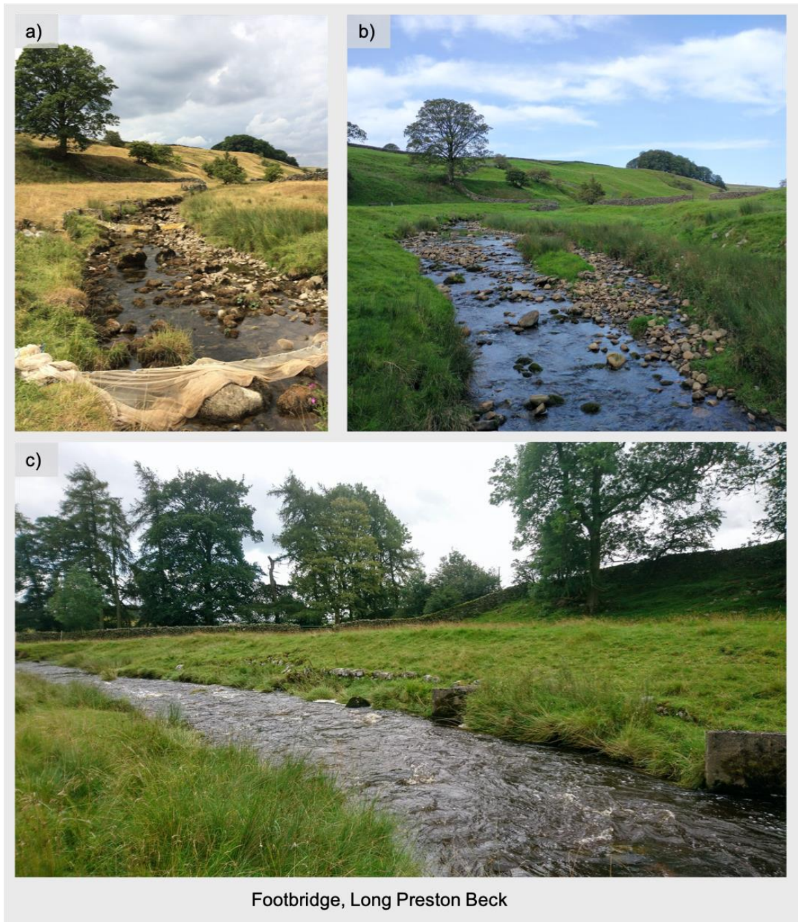
Figure 2.6 Photographs of Footbridge: a) prior to field surveys, b) normal conditions and c) moderate flow conditions.
