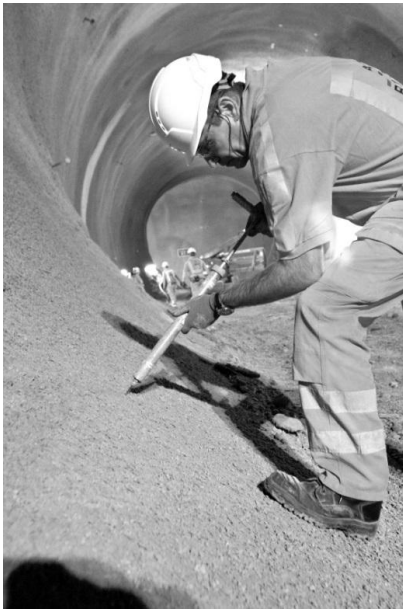
Fig. 1: Early-age assessment of sprayed concrete strength using needle penetrometer.
