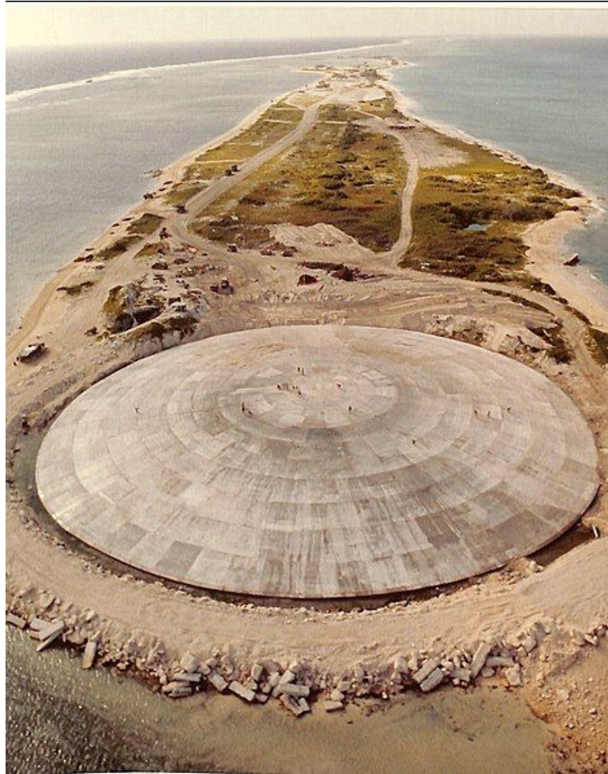
Runit Dome (or Cactus Dome), Runit Island, Enewetak Atoll . Aerial view. In 1977-1980 the crater created by the Cactus shot of Operation Hardtack I was used as a burial pit to inter 84,000 cubic meters of radioactive soil scraped from the various contaminated Enewetak Atoll islands. The image demonstrates the intersection of hyperobjects - nuclear waste and climate crisis: the dome is cracking, and increased storm surges threaten to break it open. Wikimedia Commons, Public Domain
