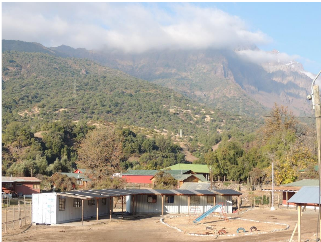
Figure 6.9. Multi-purpose containers in Chacayes.
