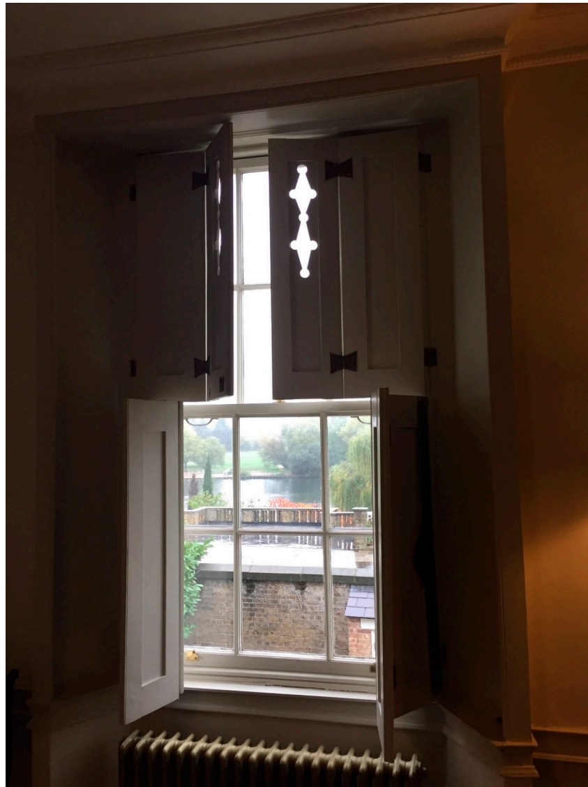
Figure 4. The vertically sliding sash window is one of the cleverest elements of building technology ever invented, allowing ventilation at different heights, and not slamming shut or open in high winds (the perennial problem of hinged casement windows). The flat profile allowed it to be used with awnings and shutters, to give the highest possible degree of control over sunlight, ventilation, and security. Sash windows arguably made the terrace house possible, which characterises townscapes of the 18th and 19th centuries. ©Robyn Pender.
