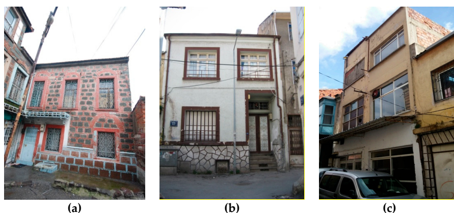
Figure 8. (a) Building 21(HR) (9% energy saving by Package 1; 60% energy saving by Package 2), (b) Building 8 (HNR) (9% energy saving by Package 1; 42% energy saving by Package 2) and (c) Building 11 (C) (44% energy saving by Package 1; 67% energy saving by Package 2) where retrofit solutions can be applied initially.
