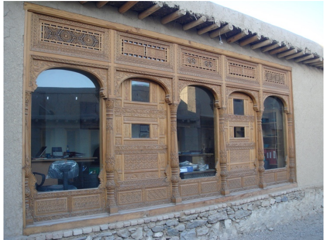
FIGURE 23 A RESTORED PANJARE (WINDOW) SCREEN AT THE TURQUOISE MOUNTAIN FORT. PHOTOGRAPH C. WYNDHAM
