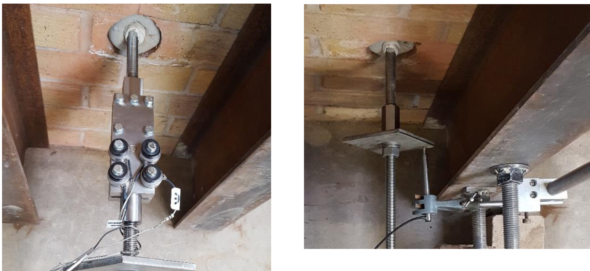
Figure 5-8 Instrumentation: a) donut load cells, b) spring LVDT
