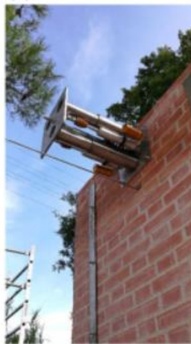
Figure 2-7 masonry wall equipped with LICORD system, credits to Giresini et al. (2021)
