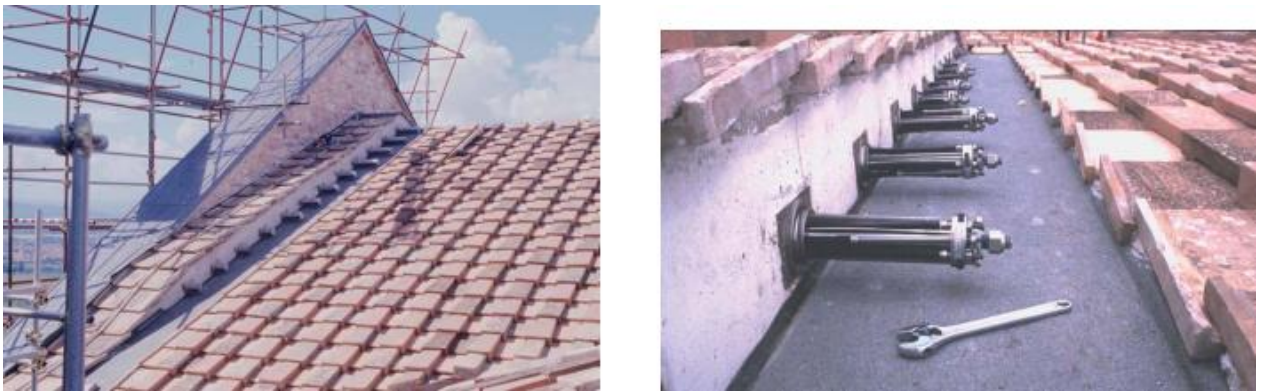
Figure 2-10. Photographs of the SMA device insertion for the Assisi Basilica tympanum (IT) (Indirli and Castellano 2008);
