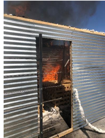
Fig. 11 d) Polycarbonate sheets almost completely melted away
