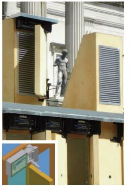
The DEI concept consists of two elements; a thermally insulating shutter that opens and closes over a window and a drive mechanism to operate it (inset). The drive mechanism is designed to open the shutter when conditions are favourable and close the shutter when it is too hot or too cold outside. The mechanism operates using the phase-change of wax, which responds to the outside temperature and heat from sunshine to melt and expand during the day and freeze and contract during the night.
