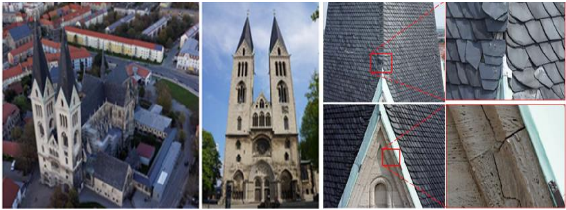
Figure 3.16: 1200-year-old Masonry cathedral with Roof and façade inspections results: Source; Hallermann and Morgenthal (2015)
