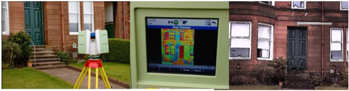
Figure 8.6: 3D laser scanning of the building façade
