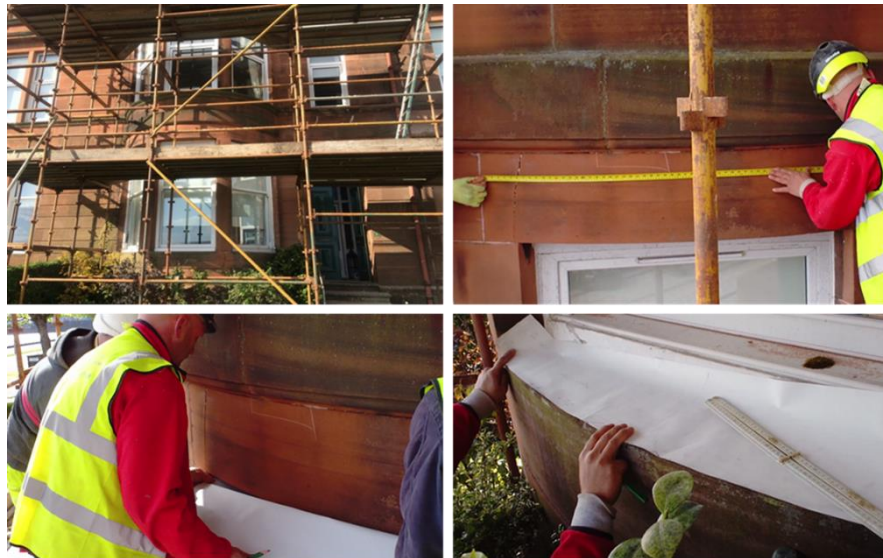
Figure 8.10: Scaffold for Conventional in-depth survey access
