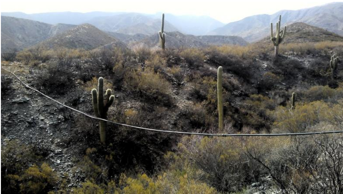
Figure 9.15: A hose of the World Bank-DCI Project suspended over a ravine near Yasyamayo (CIAV). The system worked, but the amount of water conveyed by the tube is too small as to cover all needs of the local families, the most part of which emigrated to the city. September 2018.
