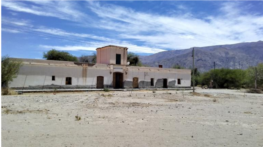
Figure 9.29: The large white house of the Chico family in El Bañado had been a missionary estate until the end of the 19 th Century when the landowners acquired it and became the centre of the exploitation of the territory. The descendants of the Chico family still own the place, which was being restored at the time of my visit to make it into a hotel on the privileged position on the Route 40. November 2018.
