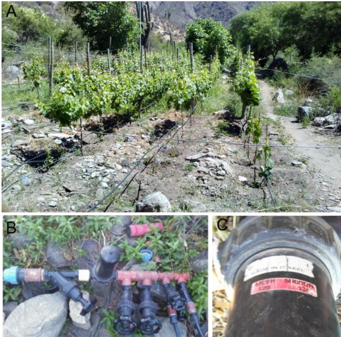
Figure 9.20: a) Vineyard served by the drip irrigation system installed through the APS-EU Project; B) and c): details of the head tap of the system, which employed Israeli technology specifically developed for extremely arid and semi-arid regions. October 2018.
