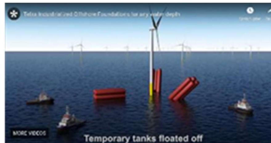
Remove temporary buoyancy after Connecting tendons
