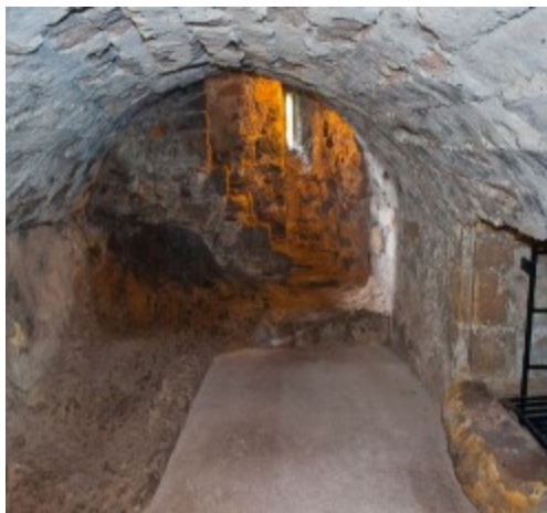
Fig. 13. Dirleton Castle. The upper prison with hatch entry to lower prison to the right of the picture.
