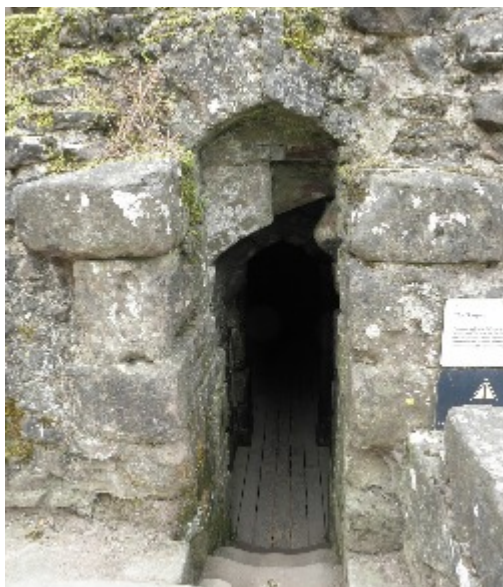
Fig. 10. Goodrich Castle. The narrow C14 entrance to the prison cell adjacent to and east of the keep. Two successive doors, both with draw-bars, controlled entry.
