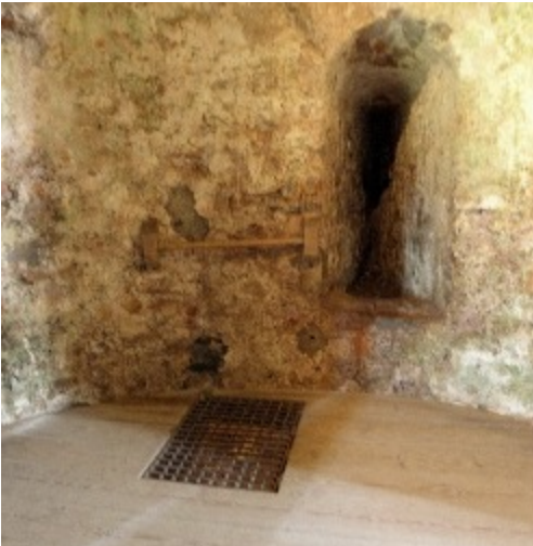
BELOW: Figs. 8, 9. Pembroke Castle. The early-mid C13 'Prison Tower' of the Inner Ward. Left: Grille hatch to basement. Right: basement. Limited light, but no latrine and no permanent stairs.
