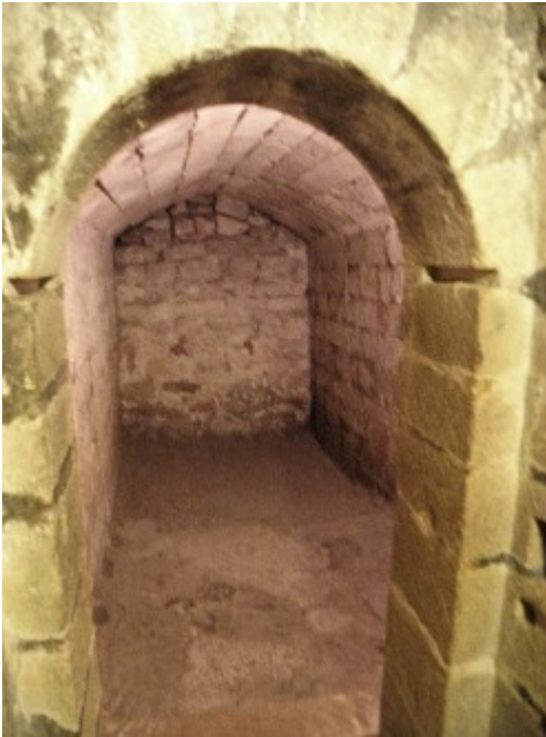
Fig. 4. Skipton Castle. Vaulted space directly below the gate-passage. Draw bar slot to right. The vaulted roof is a later insertion.
