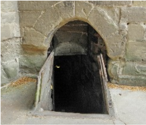
Fig. 15. Warwick. Caesar's Tower. Mid C15. Entrance to the purpose-built prison from the courtyard.
