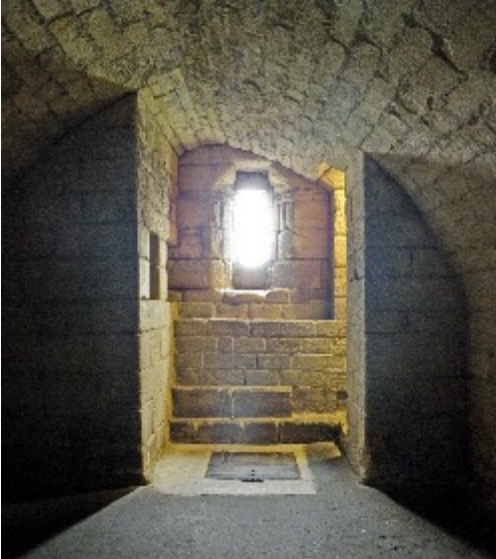
Fig 2. Warkworth Castle. Ground floor of the Great Tower (1390s). Hatch in the floor of the 'accounting room', leading to the vaulted safe or strong room below.
