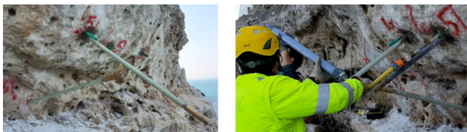
Figure 7. a) VTR bars blocked by Lampocem before injection; b) injection of MasterEmaco 222 through injection tube in CG.
