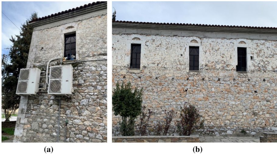
Fig. 27 Example of good quality RC ring beam which ensured connectivity of walls in a church in Tyrnavos
