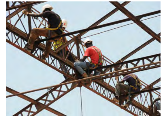
Left: local skills were used during the restoration process
