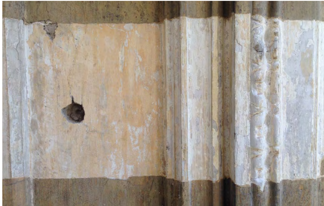
Cleaned test section showing through-colour plasters – the completed cleaning and repair.
