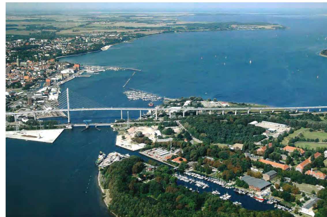
The medieval walled city (top left) is flanked by the Baltic, islands, a commercial port and modern housing located away from the heart of the city.
