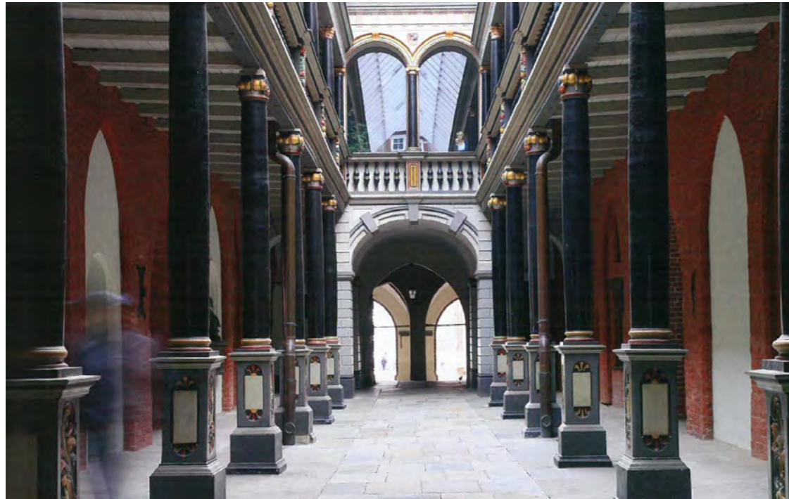
A glass roof and glazed infill was added to the 17th Century open courtyard and gallery and the columns and decoration over-painted in the 1980's.
