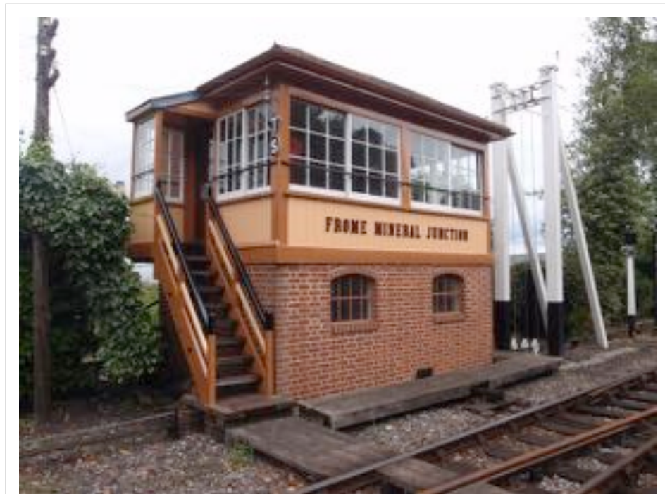
Figure A.50: Frome Mineral Junction Signal Box as relocated to the Great Western Society at Didcot. (Author 2016)
