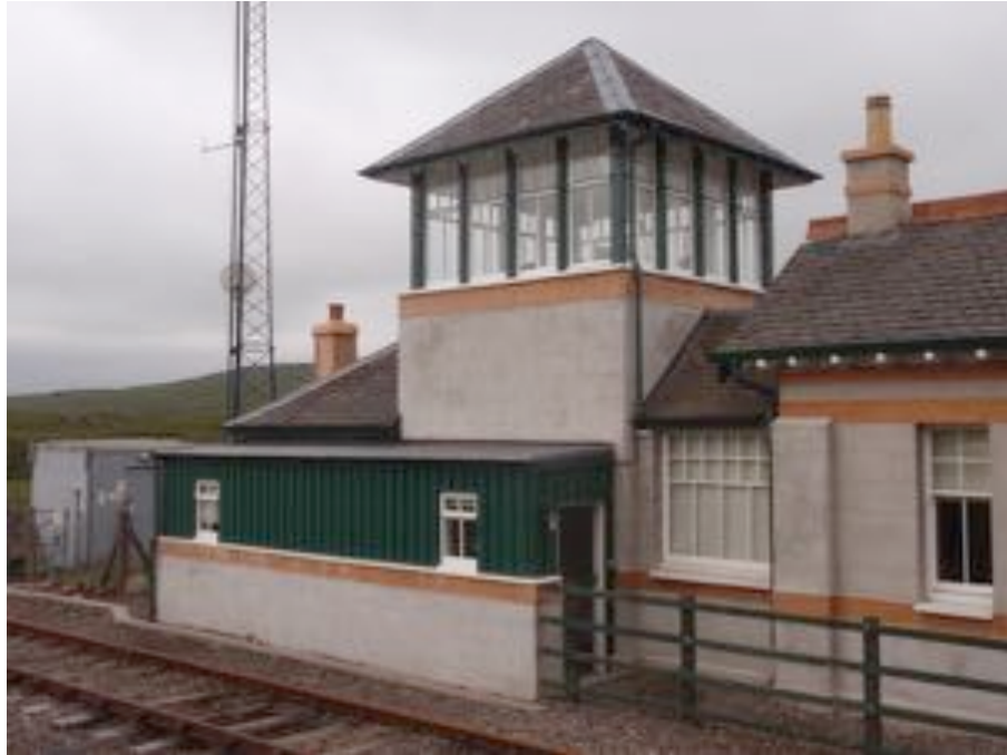
Figure A.34: Corroul Signal Box. (Author 2018)
