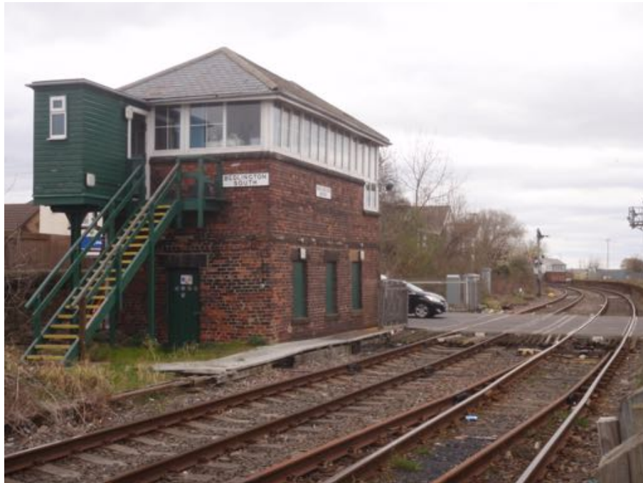
Figure A.9: Bedlington South Signal Box. Visible in the distance is Bedlington North Signal Box, illustrating the close co-location of signal boxes at formerly busy locations. (Author 2019)
