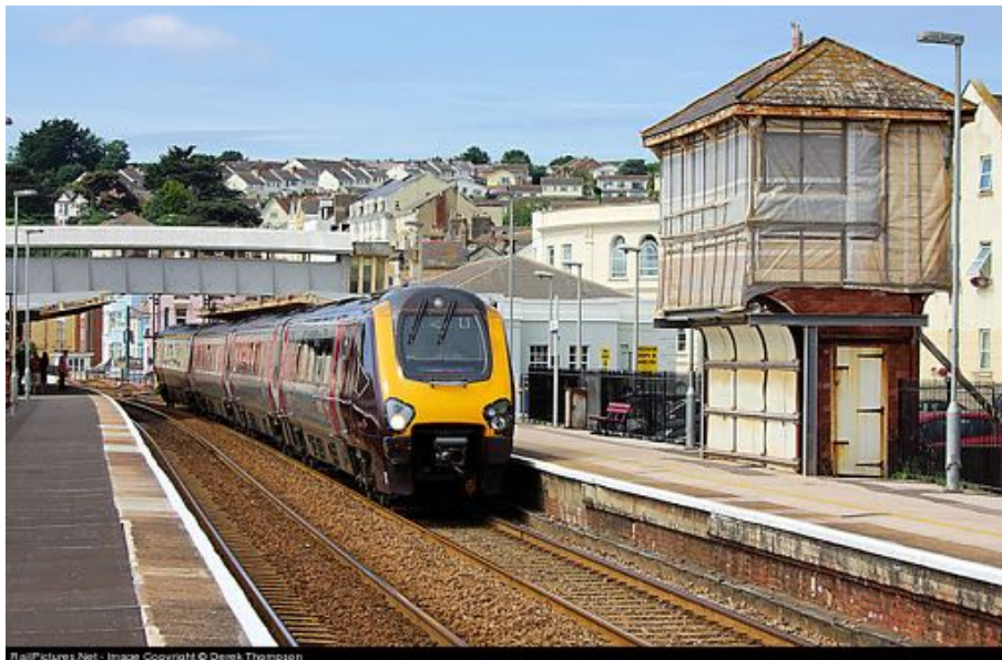
Figure 3.6: Dawlish Signal Box, tentatively conserved against the coastal environment, seen shortly before demolition. (Thompson, D. 2013, used with permission)
