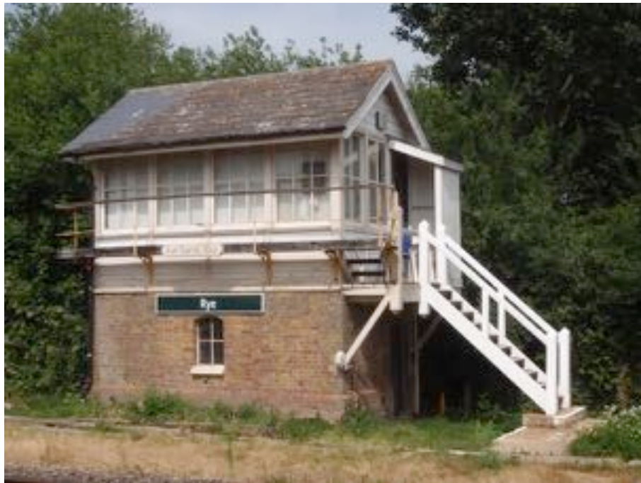
Figure A.110 Rye Signal Box. (Author 2018)
