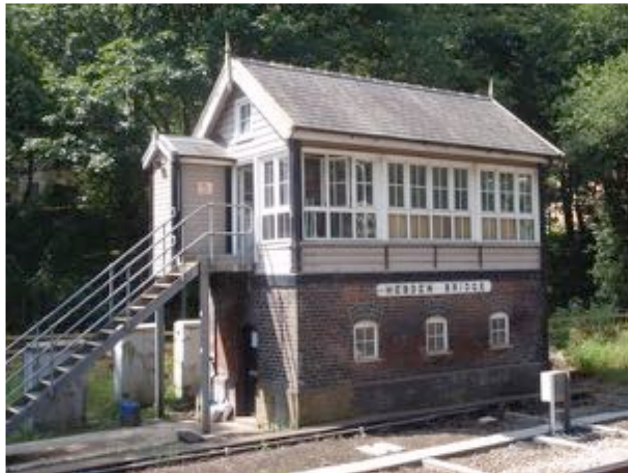
Figure A.59: Hebden Bridge Signal Box. (Author 2018)
