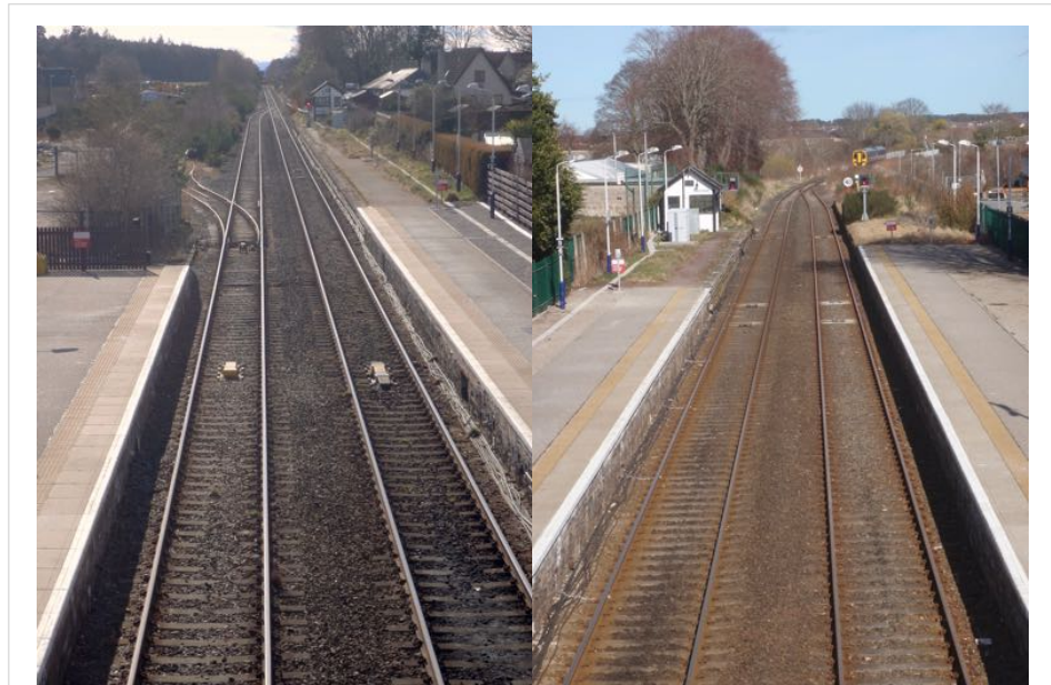
Figure 6.5: See from the station footbridge, platform end Nairn West (left, far end right hand platform) and Nairn East (right, far end left hand platform). (Author 2018)
