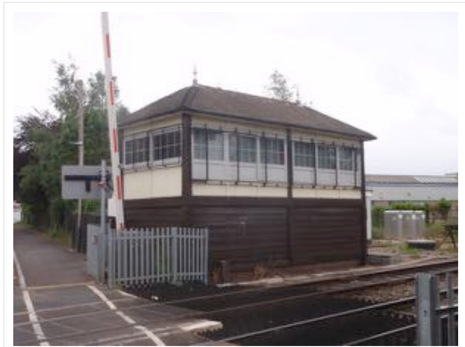
Figure A.4: Alstone Crossing Signal Box. (Author 2018)
