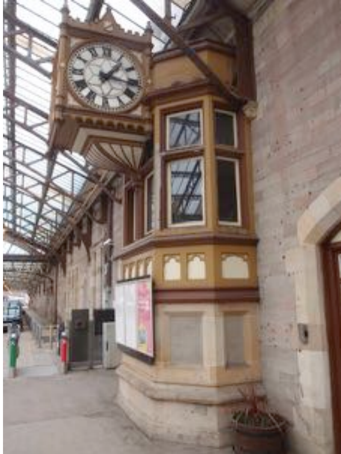
Figure A.96: Perth Down Centre Signal Box. (Author 2018)
