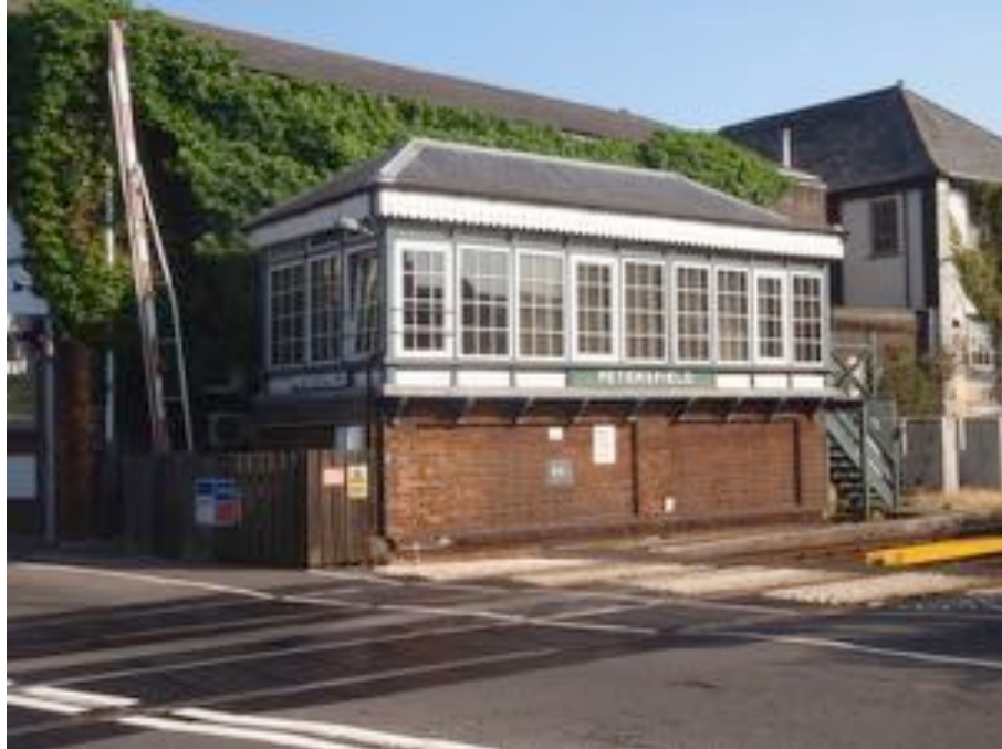
Figure A.97: Petersfield Signal Box. (Author 2018)
