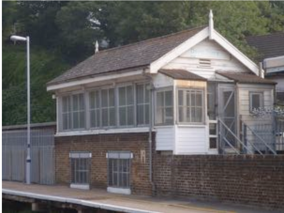
Figure A.40: Dover Priory Signal Box. (Author 2018)
