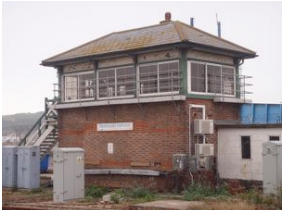
Figure A.89: Newhaven Harbour Signal Box. (Author 2016)
