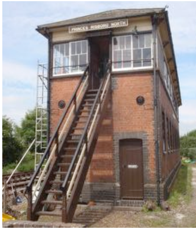
Figure A.101a: Princes Risborough North Signal Box. (Author 2018)
