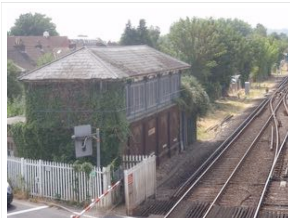
Figure A.58: Havant Junction East Signal Box. (Author 2018)
