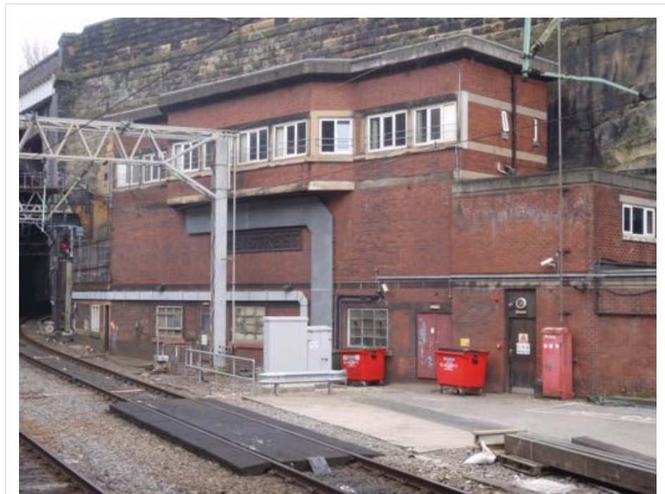
Figure A.73: Liverpool Lime Street Signal Box. (Author 2016)
