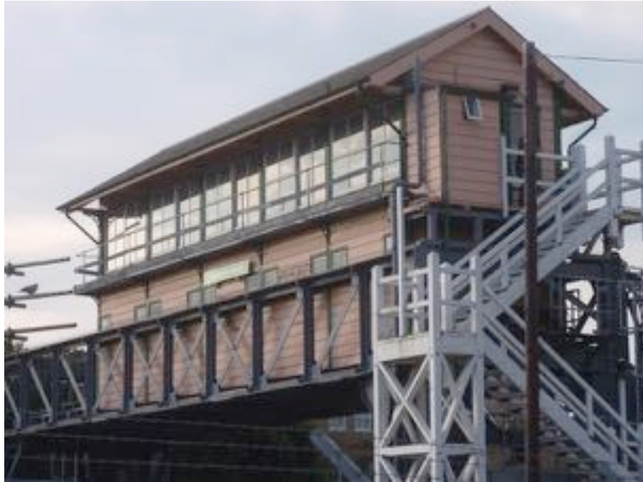
Figure A.25: Canterbury West Signal Box. (Author 2018)
