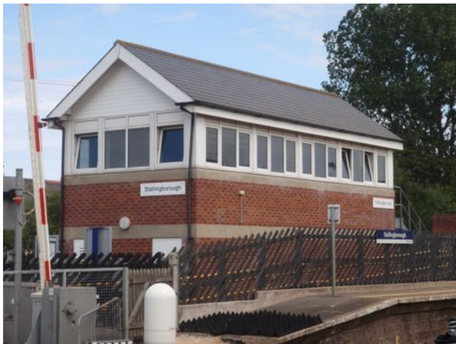
Figure A.119: Stallingborough Signal Box. (Author 2015)
