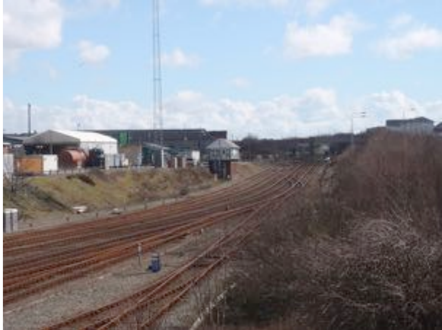
Figure A.63: Holyhead Signal Box. (Author 2016)
