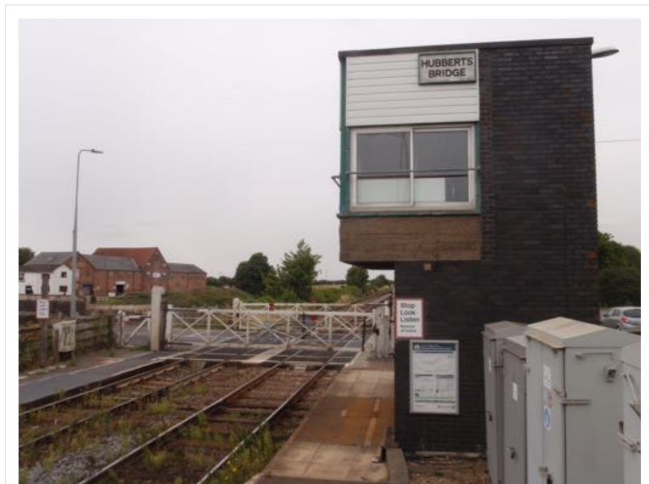
Figure 6.4: Hubberts Bridge Signal Box, with main road to right and commercial property the other side of South Forty Foot Drain bridged left of the level crossing. (Author 2016)
