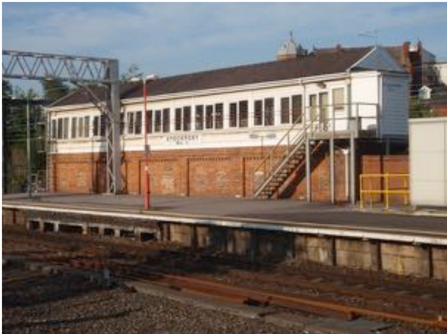
Figure A.122: Stockport No 1 Signal Box. (Author 2018)
