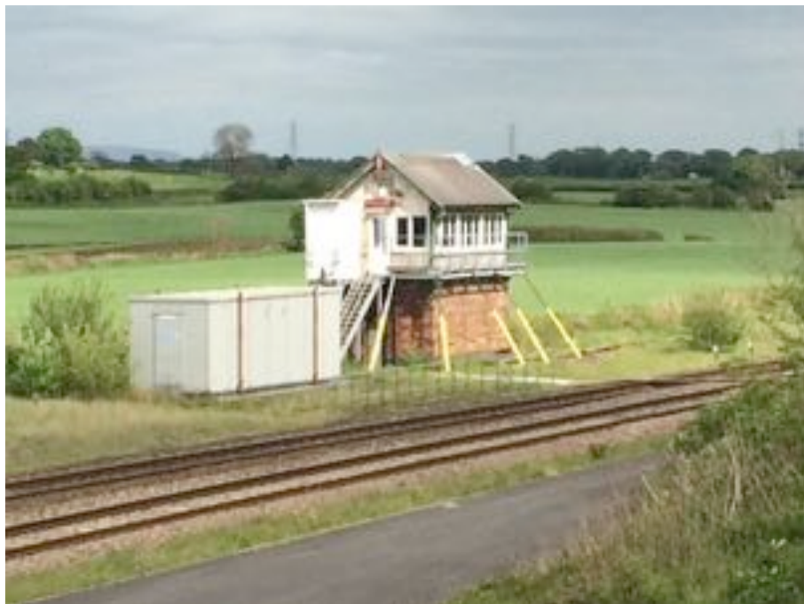
Figure A.112: Salwick No 2 Signal Box. (Author 2016)
