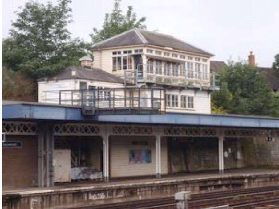
Figure A.16: Bournemouth Central Signal Box. (Author 2016)
