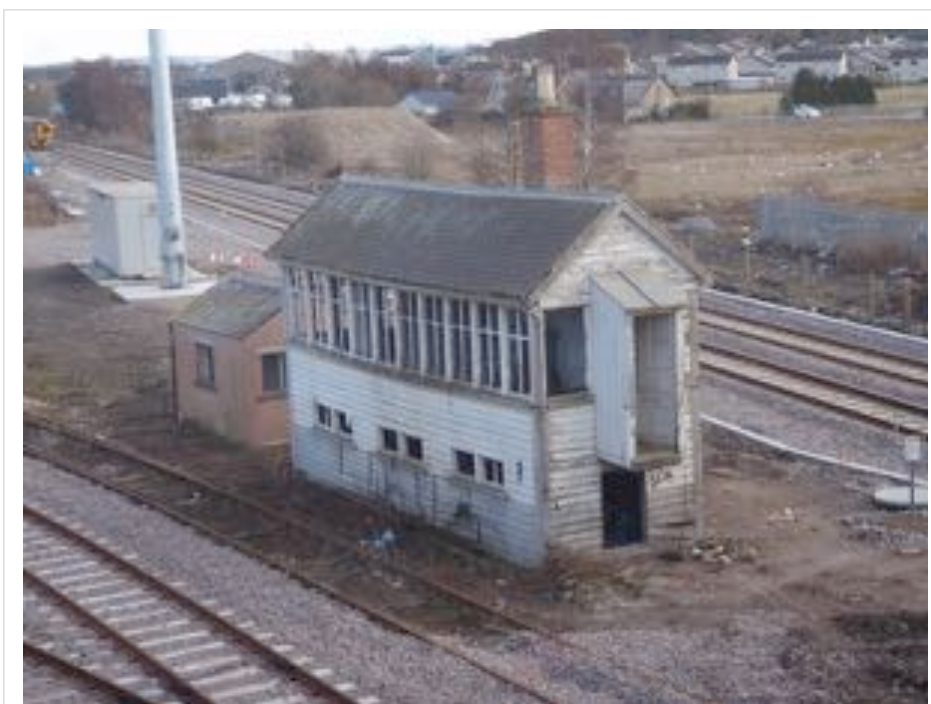
Figure A.45: Elgin Centre Signal Box. (Author 2018)
