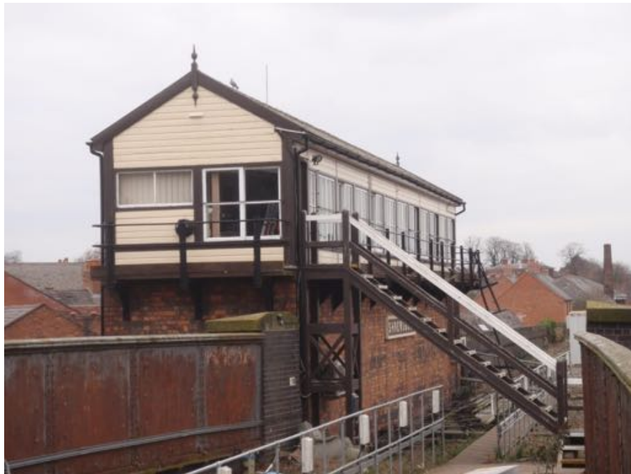
Figure A.116a: Shrewsbury Crewe Junction Signal Box as seen from Shrewsbury Railway Station. (Author 2016)
