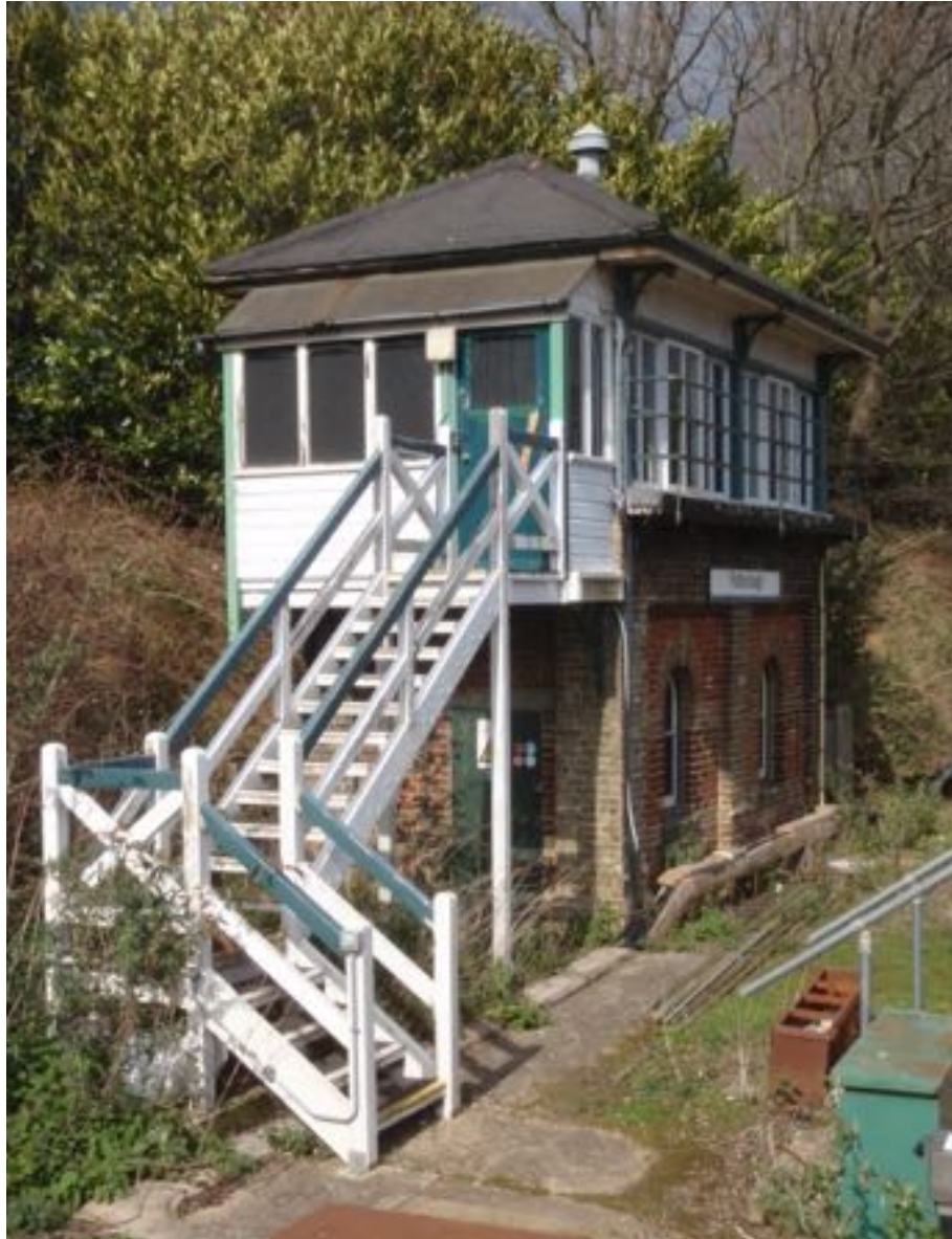
Figure A.102a: Pulborough Signal Box. (Author 2016)
