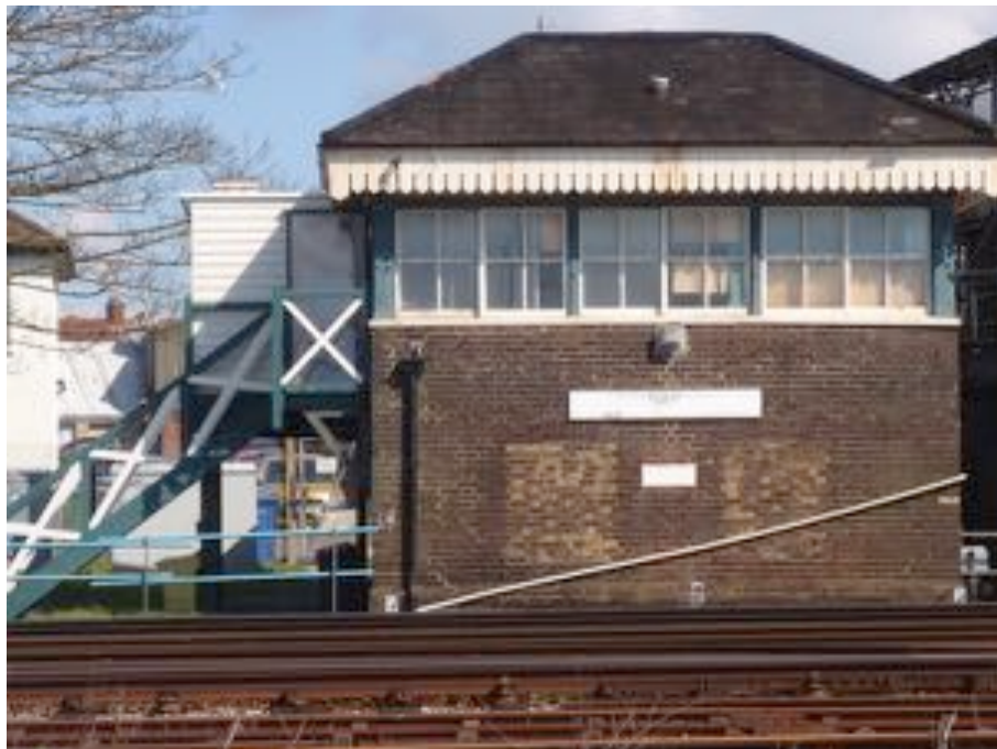
Figure A.72: Littlehampton Signal Box. (Author 2016)
