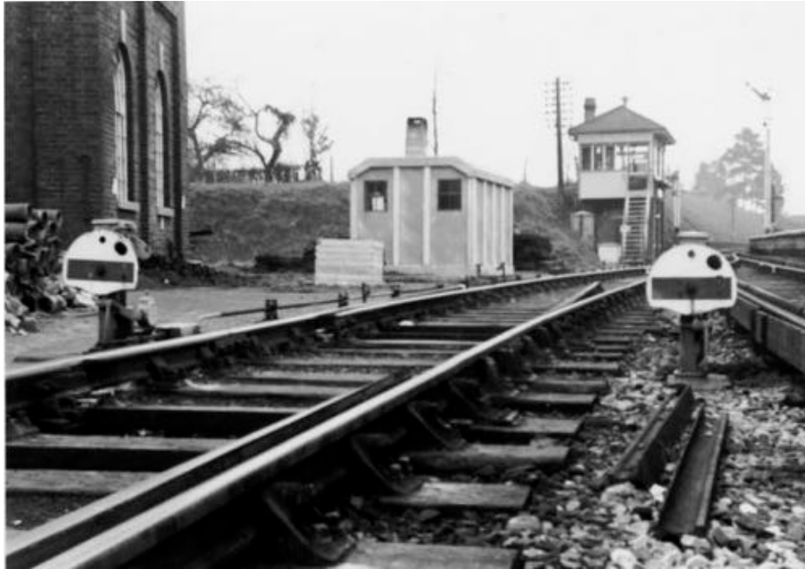
Figure A.102b: Pulborough Signal Box. Seemingly taken in 1938 after electrification of the Arun Valley main line, this photo shows the original context, with goods yard and bay platform for Midhurst branch line. This photo provides evidence of the porch addition before 1938. (Photo unknown, used by permission of Adrian Vaughan Collection)
