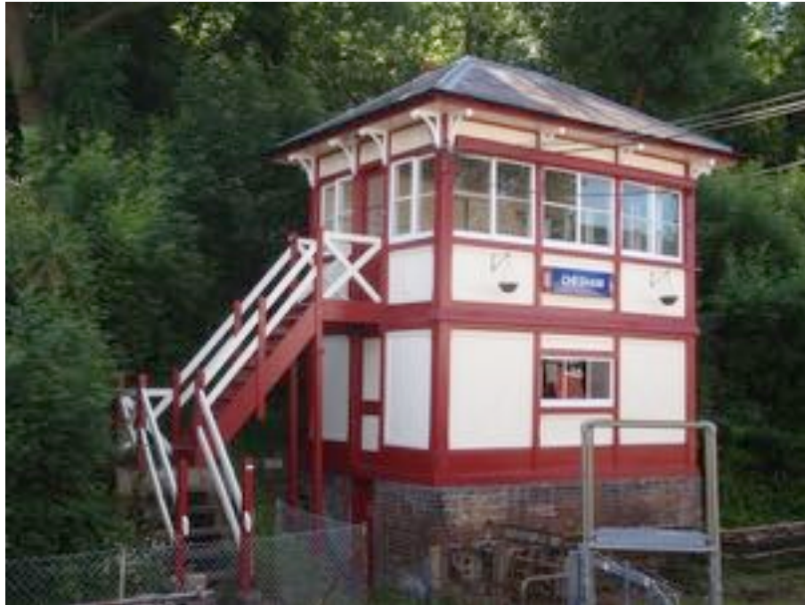
Figure A.31: Chesham Signal Box. (Author 2018)
