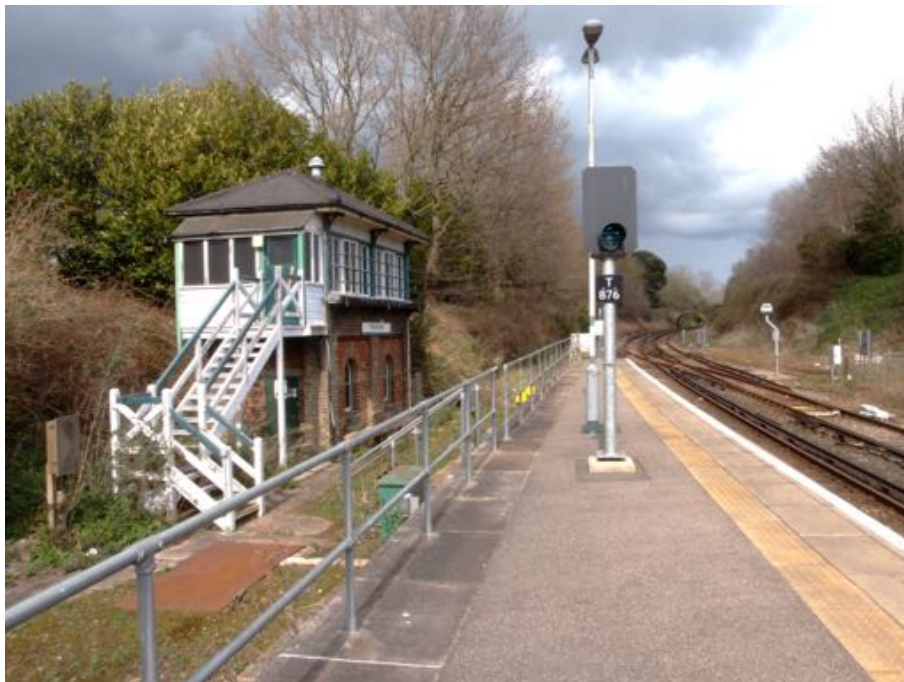
Figure 7.1: Pulborough Signal Box within the context of closed facilities and separate from modern operational railway. (Author 2016)
