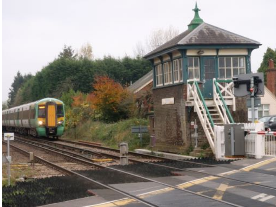
Figure 6.5: Plumpton Signal Box, showing some of the controversial replacement level crossing equipment and trackside control equipment. (Author 2016)
