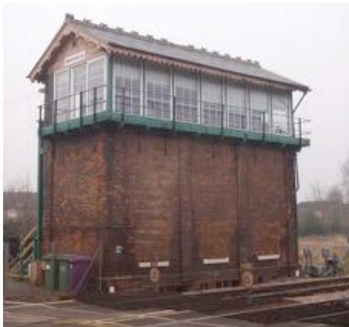
Figure A.81a: March East Junction Signal Box. (Author 2018)
