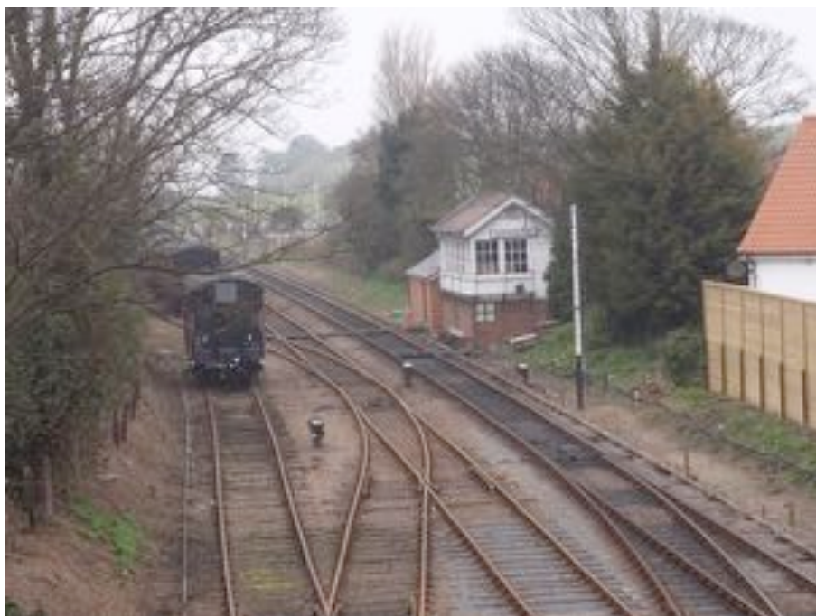
Figure A.115: Sheringham West (Wensum Junction) Signal Box. (Author 2018)
