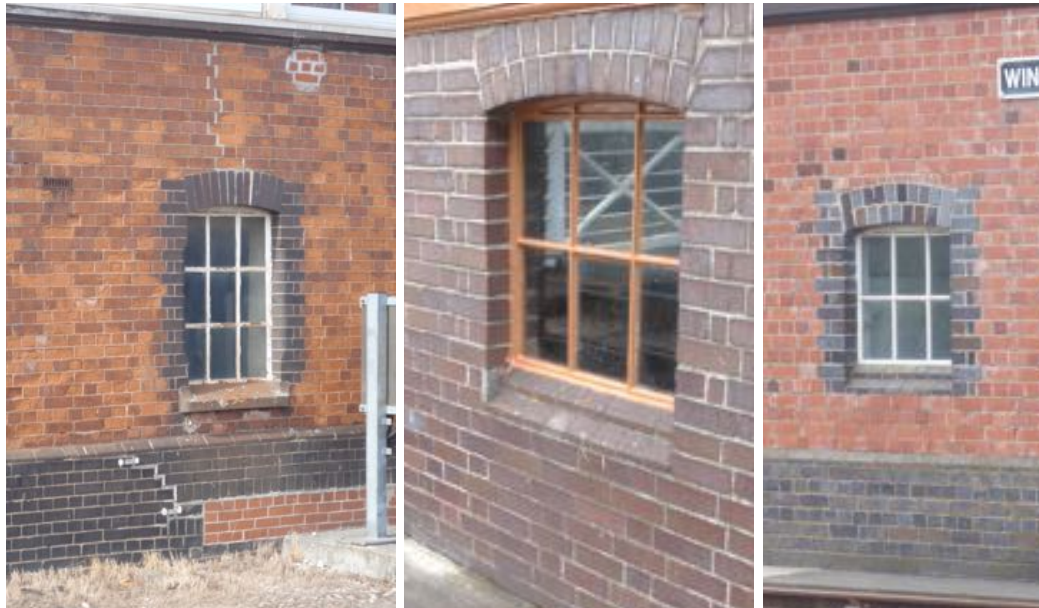
Figure 7.2: Left to right comparison of original brickwork at Truro East to replica brickwork for relocated Radstock North and reconstructed brickwork for relocated Winchcombe. (Author 2016-8)
