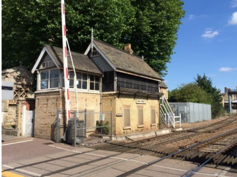
Figure A.70: Lincoln High Street Signal Box. (Author 2015)
