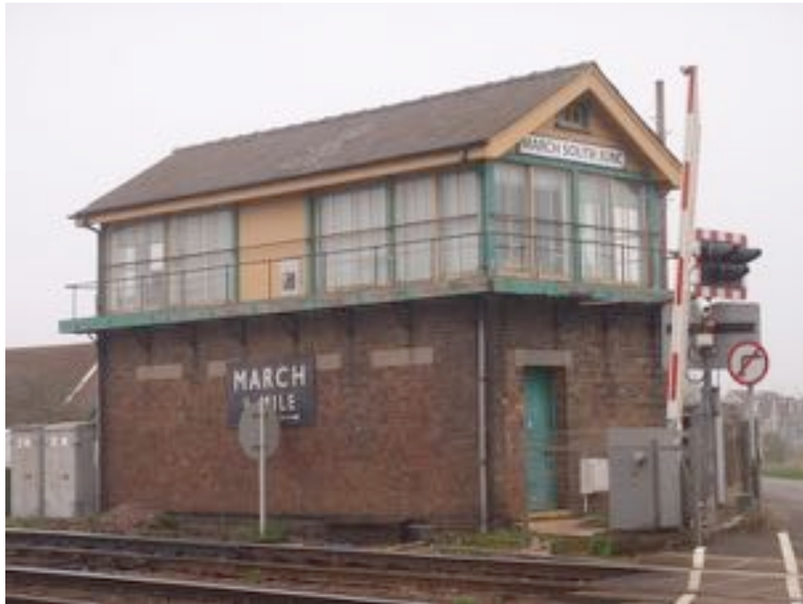
Figure A.82: March South Junction Signal Box. (Author 2018)
