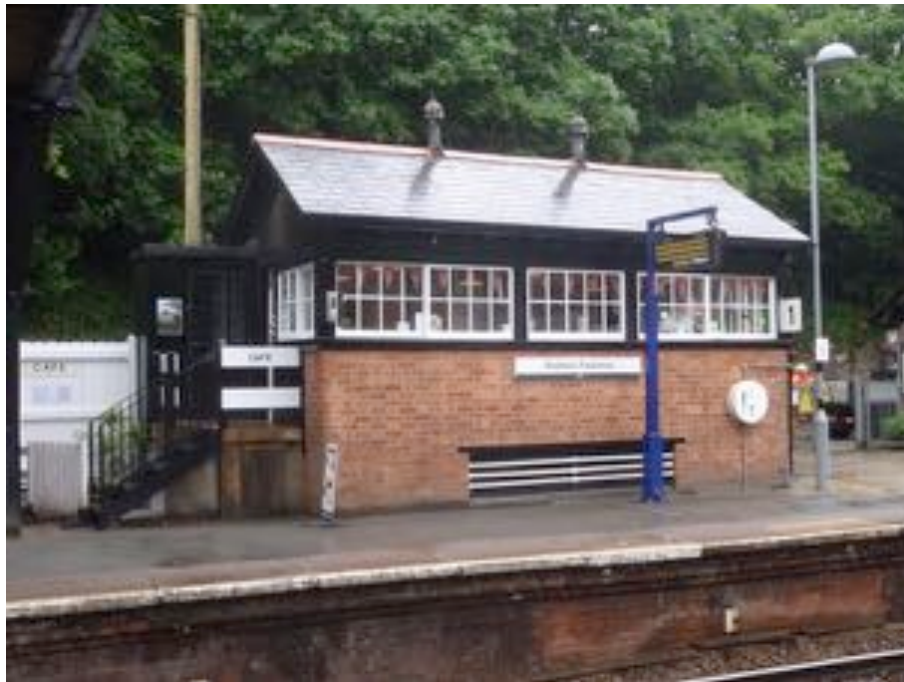
Figure A.13: Bodmin Parkway (formerly Bodmin Road) Signal Box. (Author 2018)
