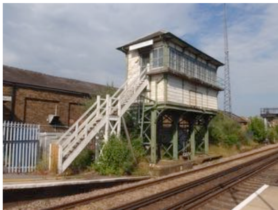
Figure A.24: Canterbury East Signal Box. (Author 2018)
