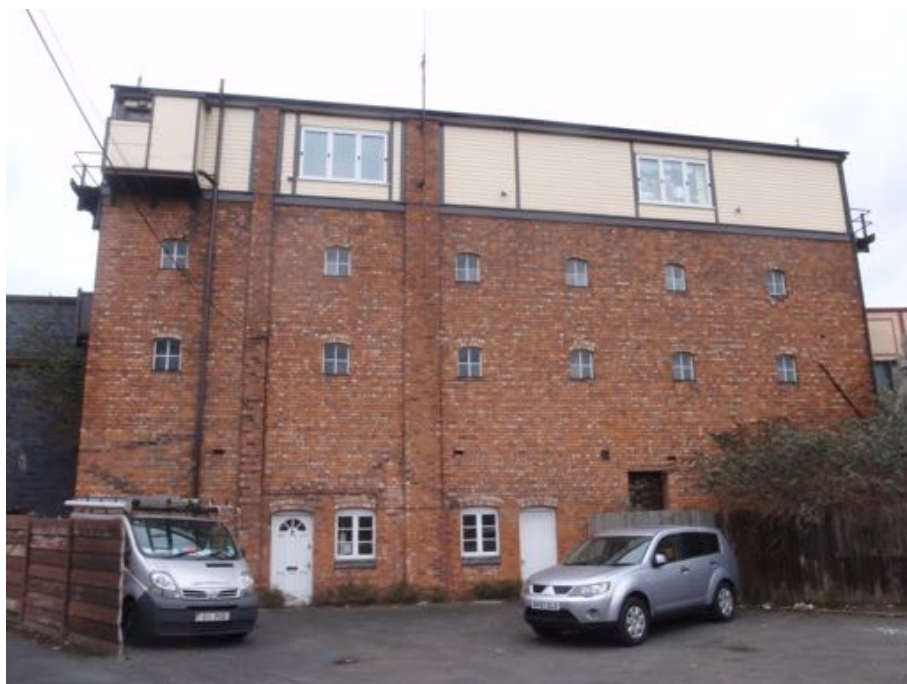
Figure A.116b: Shrewsbury Crewe Junction Signal Box as seen from street level. (Author 2016)
