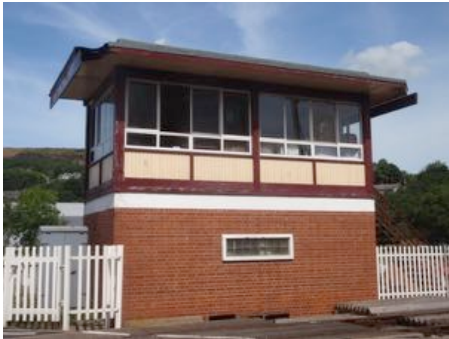
Figure A.105: Rawtenstall West Signal Box. (Author 2018)
