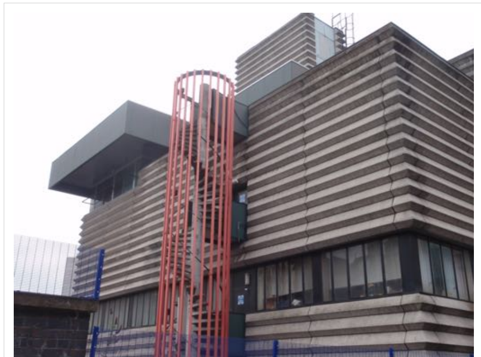
Figure 6.2: Details of cladding, deep fascia and fire escape, Birmingham New Street PSB. (Author 2016)
