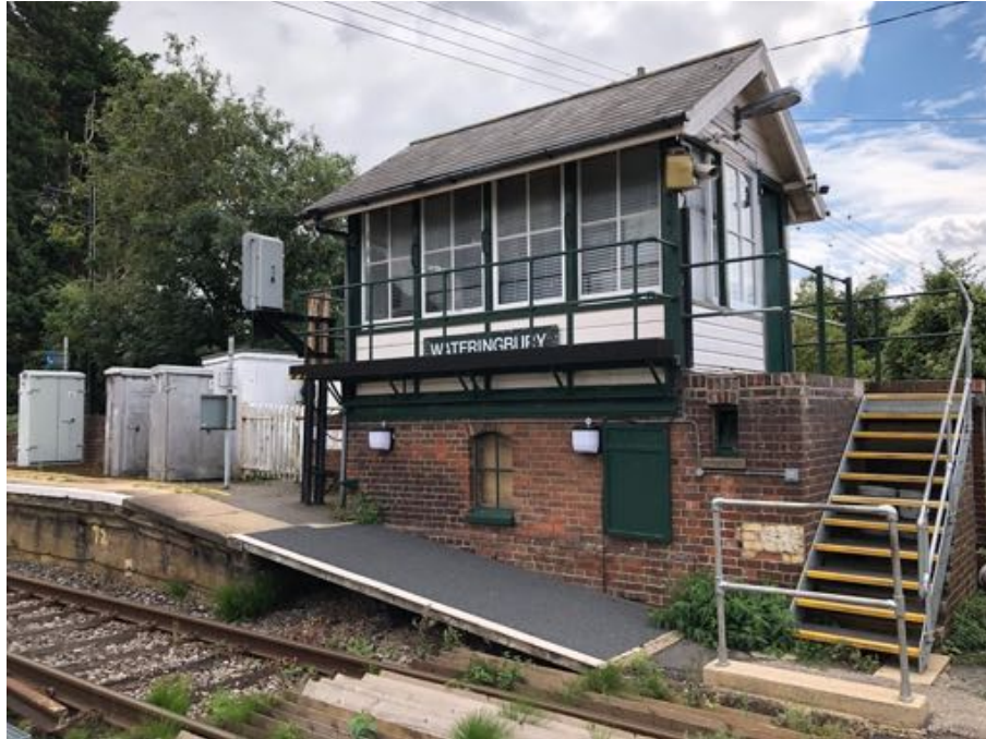
Figure A.138: Wateringbury Signal Box. (Reeves, L., 2018)
