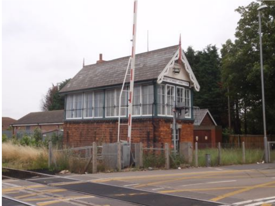
Figure A.139: West Street Junction Signal Box. (Author 2015)
