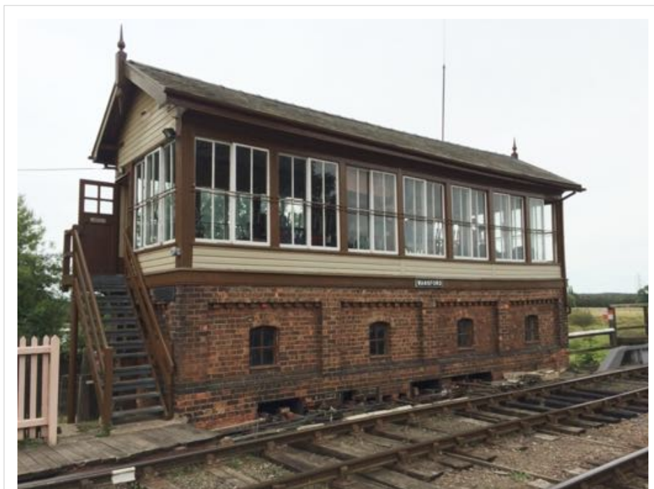
Figure A.137: Wansford Signal Box. (Author 2015)
