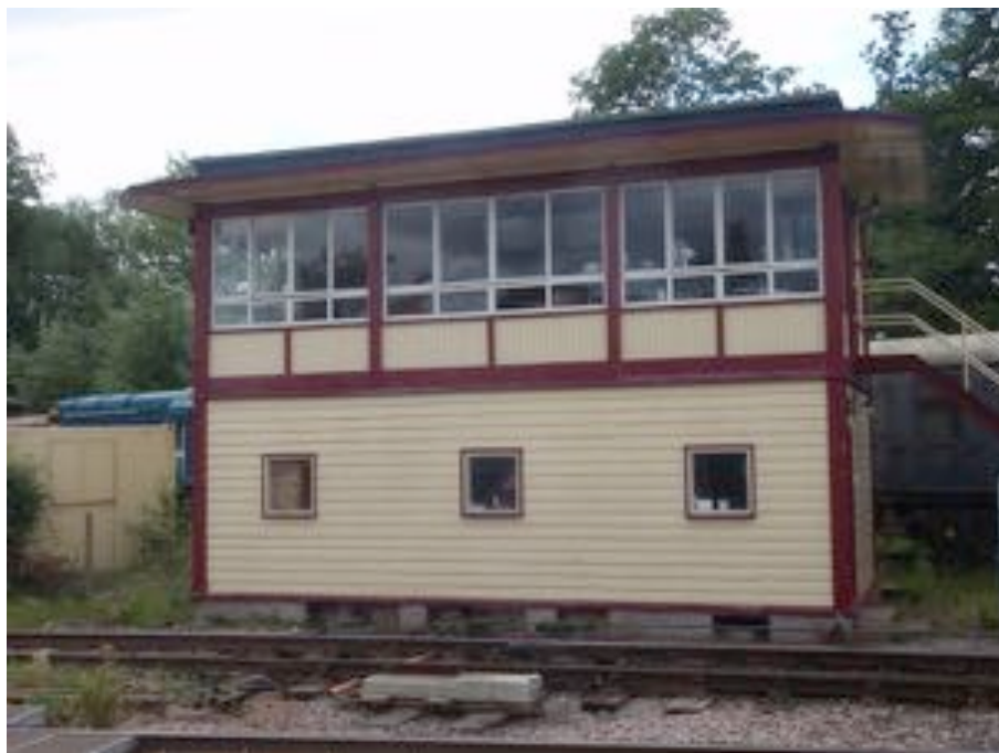
Figure A.78: Lydney Junction (Heysham Harbour) Signal Box. (Author 2017)
