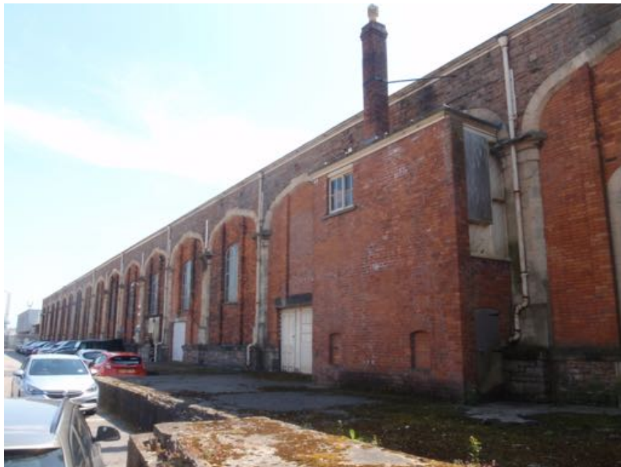
Figure A.17b: Rear of Bristol Old Station Signal Box, showing the awkward insertion into the station building. (Author 2018)
