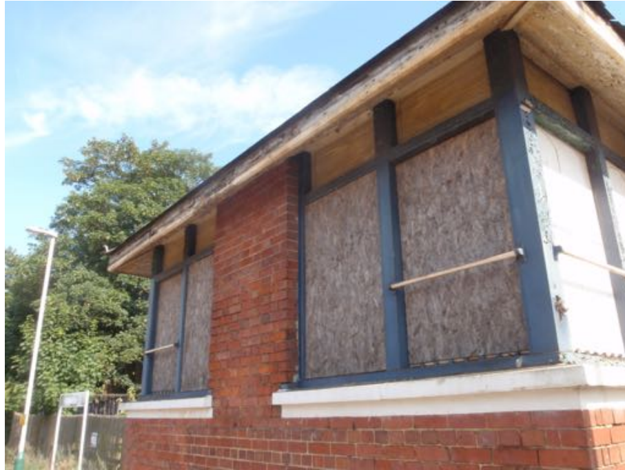
Figure 4.3: Applied protection to windows and doors, Woolston Signal Box. (Author 2018)
