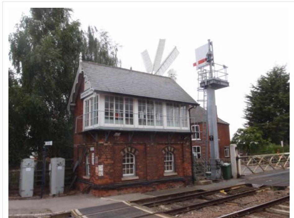
Figure A.60: Heckington Signal Box. (Author 2015)
