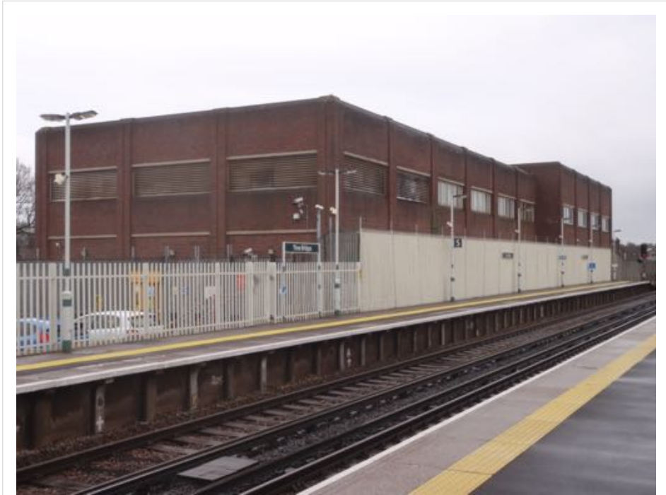
Figure A.127: Three Bridges ASC. (Author 2016)
