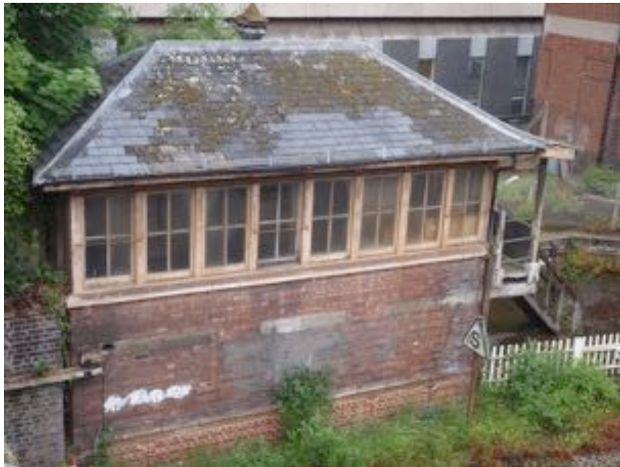
Figure A.46: Exeter Central Signal Box. (Author 2018)
