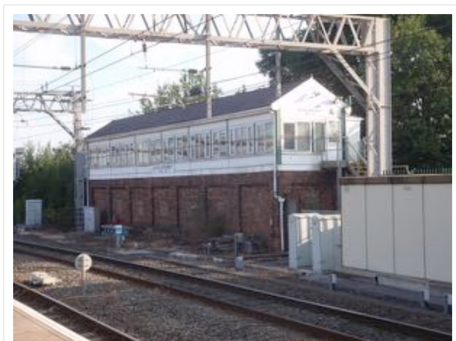
Figure A.123: Stockport No 2 Signal Box. (Author 2018)
