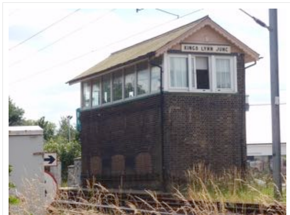
Figure A.66: Kings Lynn Junction Signal Box. (Author 2016)
