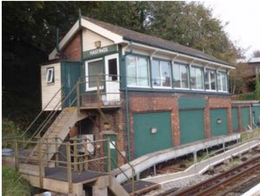
Figure A.57: Hastings Signal Box. (Author 2017)
