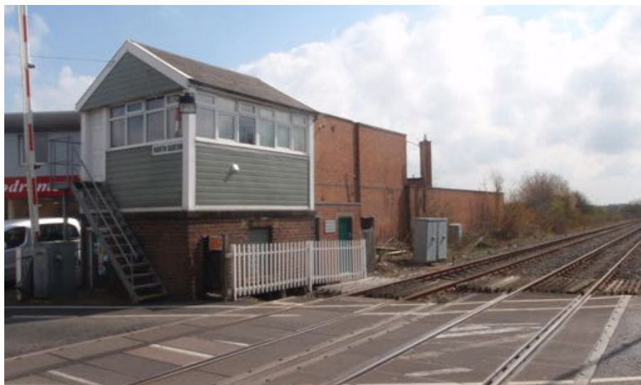
Figure A.92a: North Seaton Signal Box. (Author 2019)
