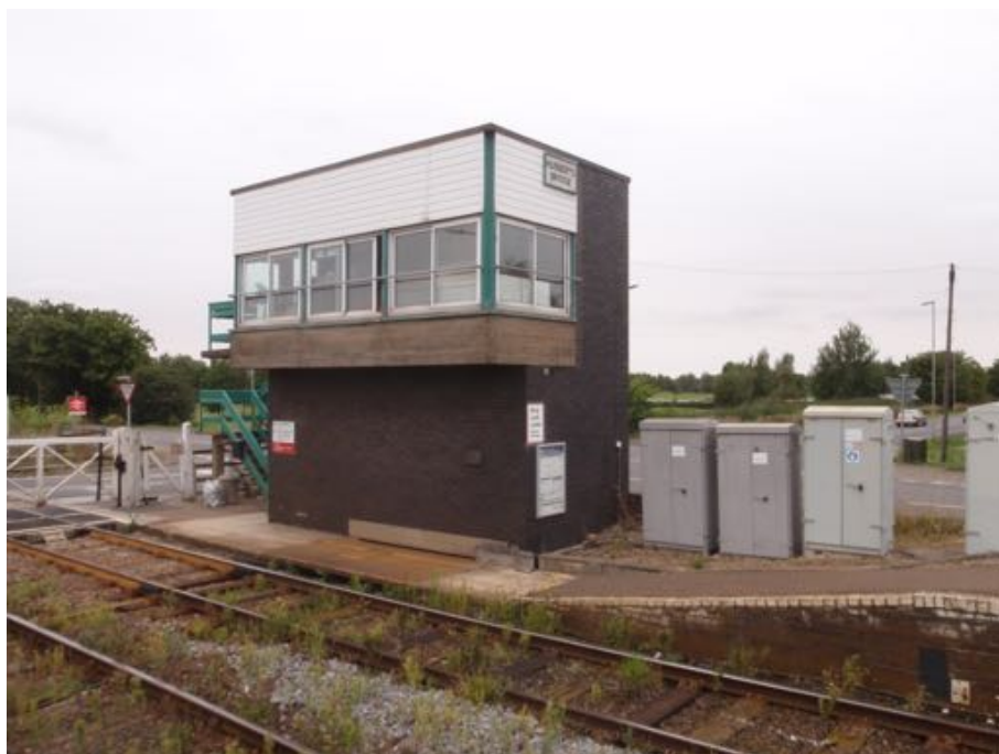
Figure A.65: Hubberts Bridge Signal Box. (Author 2015)
