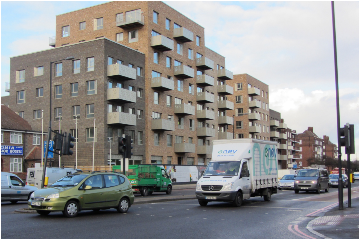
Figure 2: New social housing on a main road
