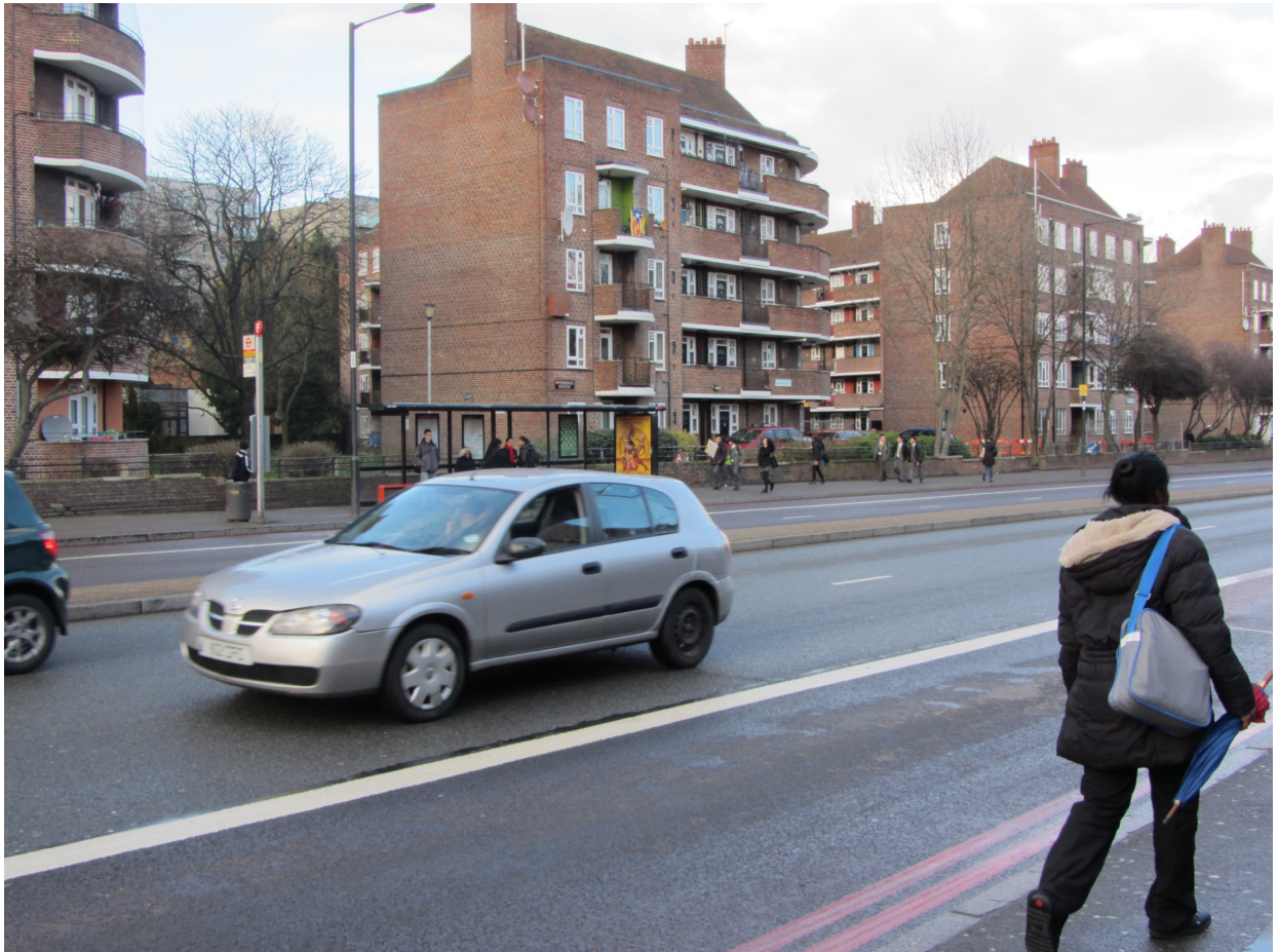
Figure 1: Some of the remaining original blocks on the estate
