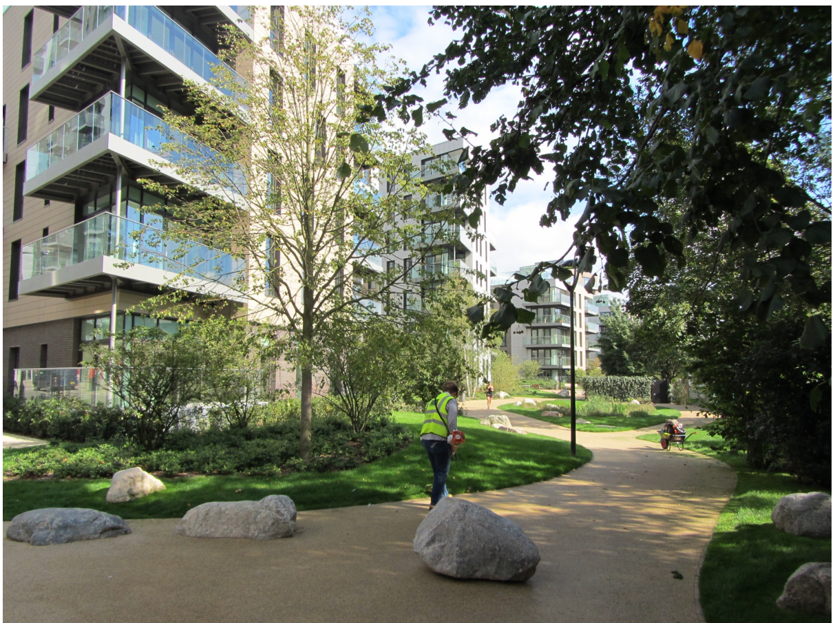
Figure 3: New private homes in a favoured location adjacent to the East Reservoir
