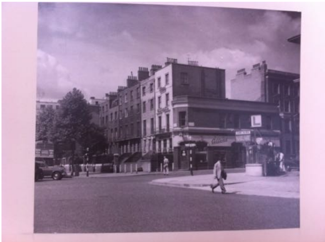
Fig. 6.5 Marylebone Road at the corner of Gloucester Place, with terraced houses and public house, 1930s (City of Westminster Archive)
