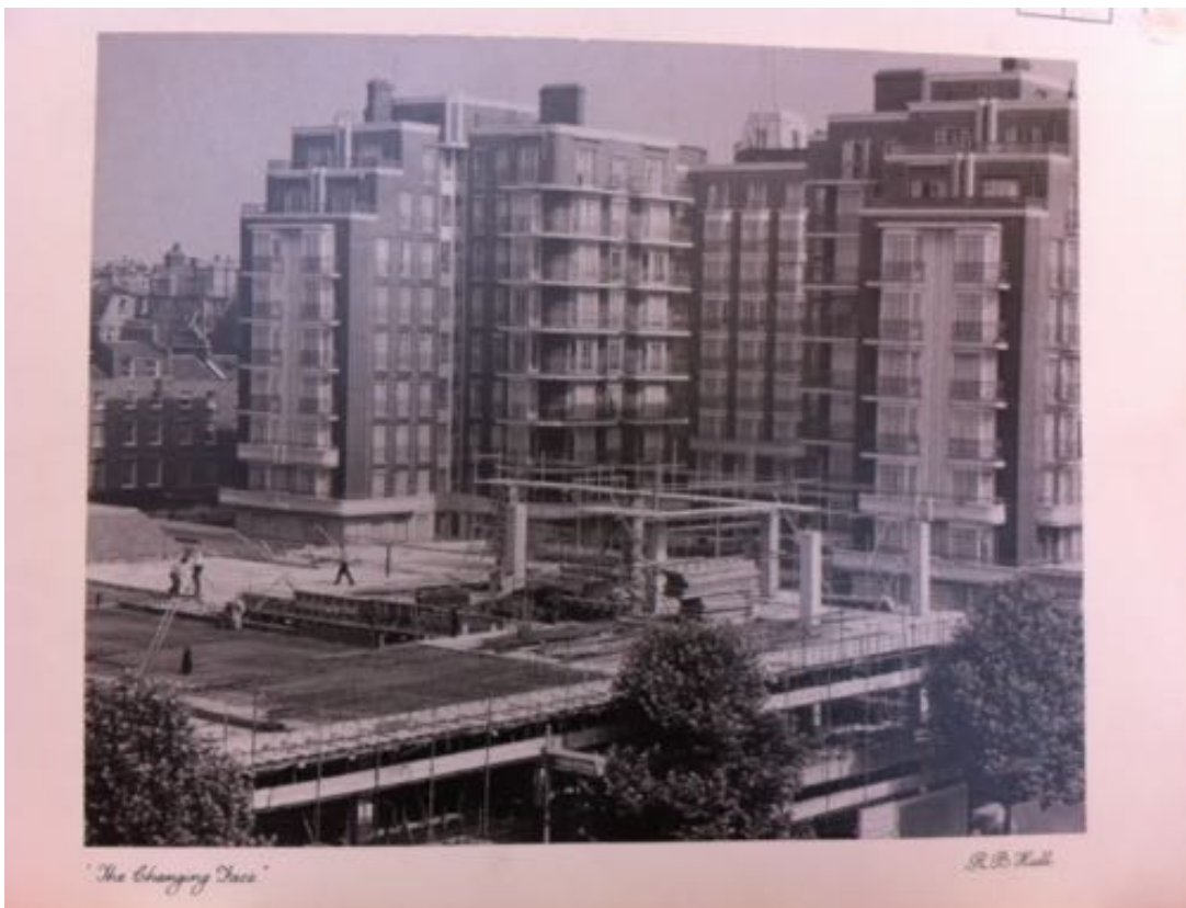
Fig. 6.13 'The Changing Face' – Erection of Castrol House, 1958 (City of Westminster Archive)
