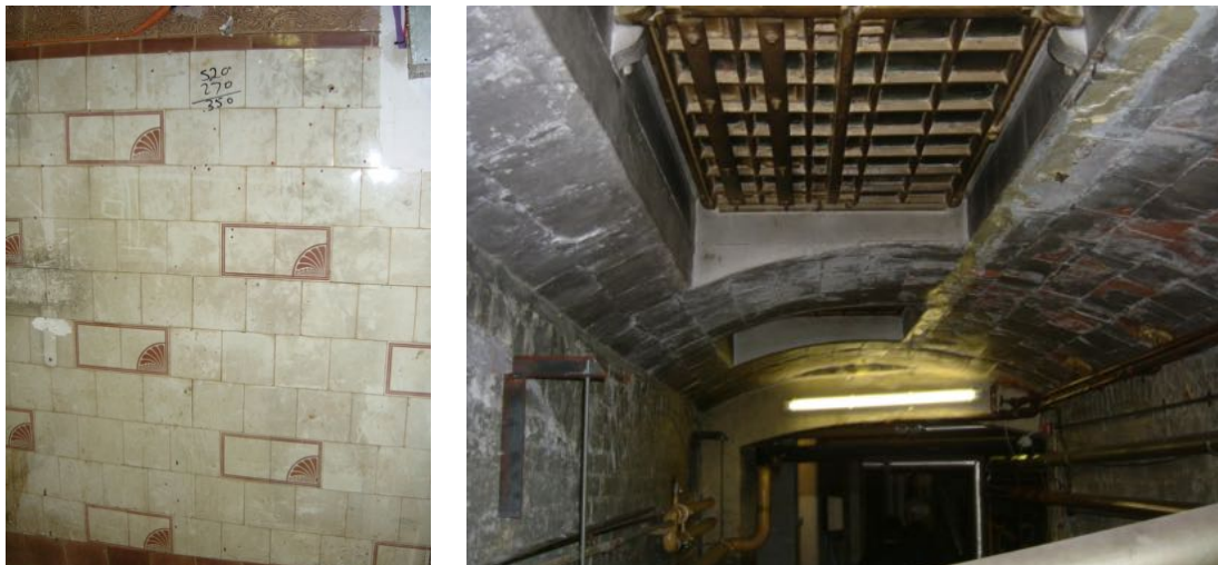
Fig. 8.10 Marylebone Magistrates Court's converted pool interiors (SMS site visit 23 November 2006)
