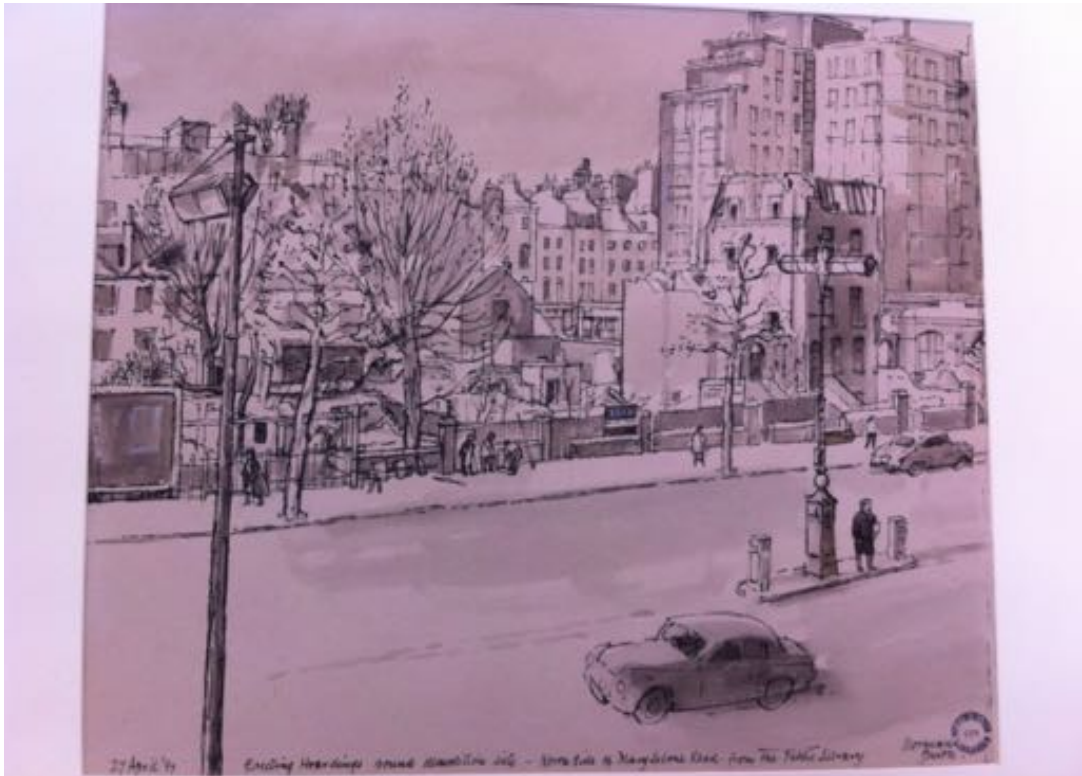
Fig. 6.12 Sketch recording demolition, 1957 (City of Westminster Archive)
