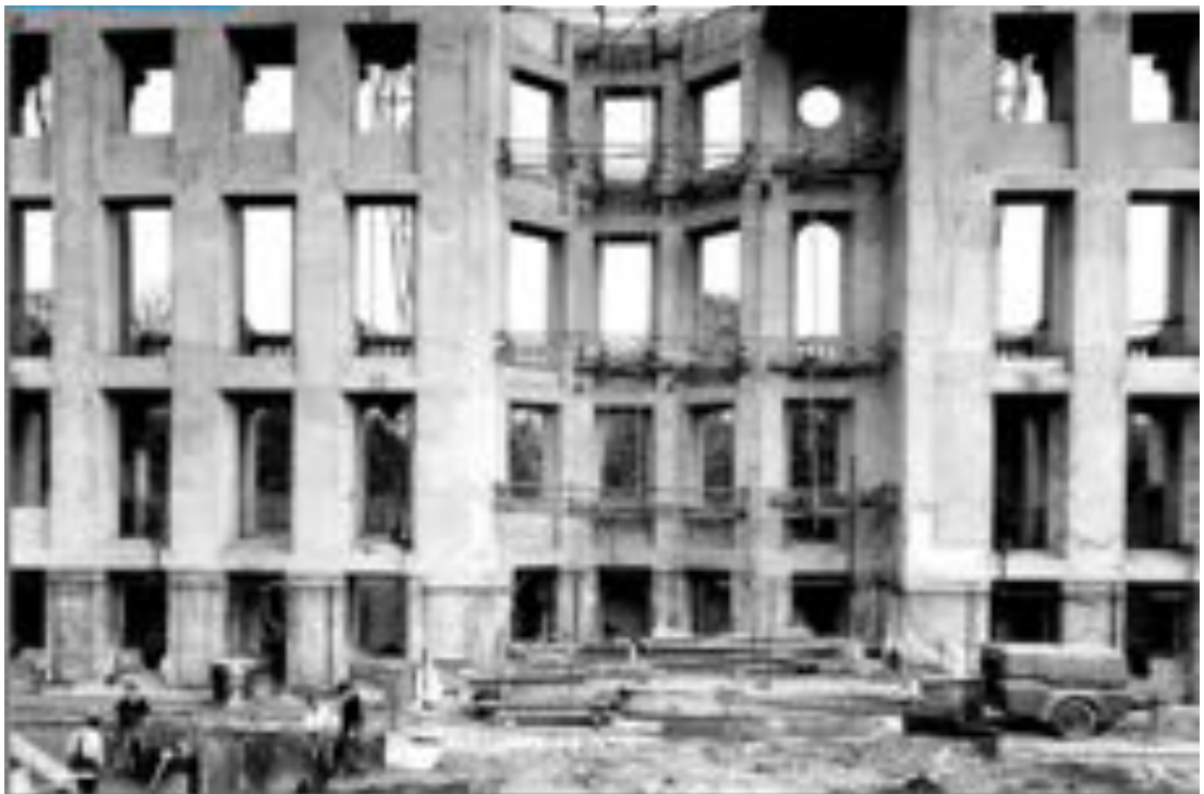
Fig. 5.7 Sussex Place, Regent's Park, condition in the 1950s (Copyright Crown Estates)
