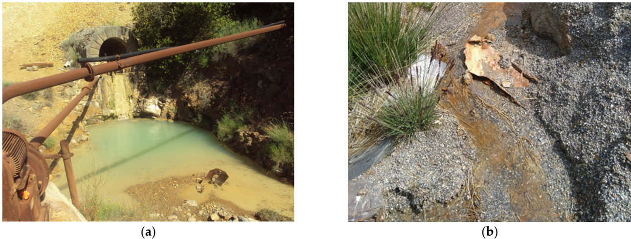
Figure 1. (a) Example of a drainage adit in the Montevecchio mine district (south-west Sardinia, Italy); (b) leachate from tailings heaps in Nant y Mwyn lead mine (central Wales, UK).
