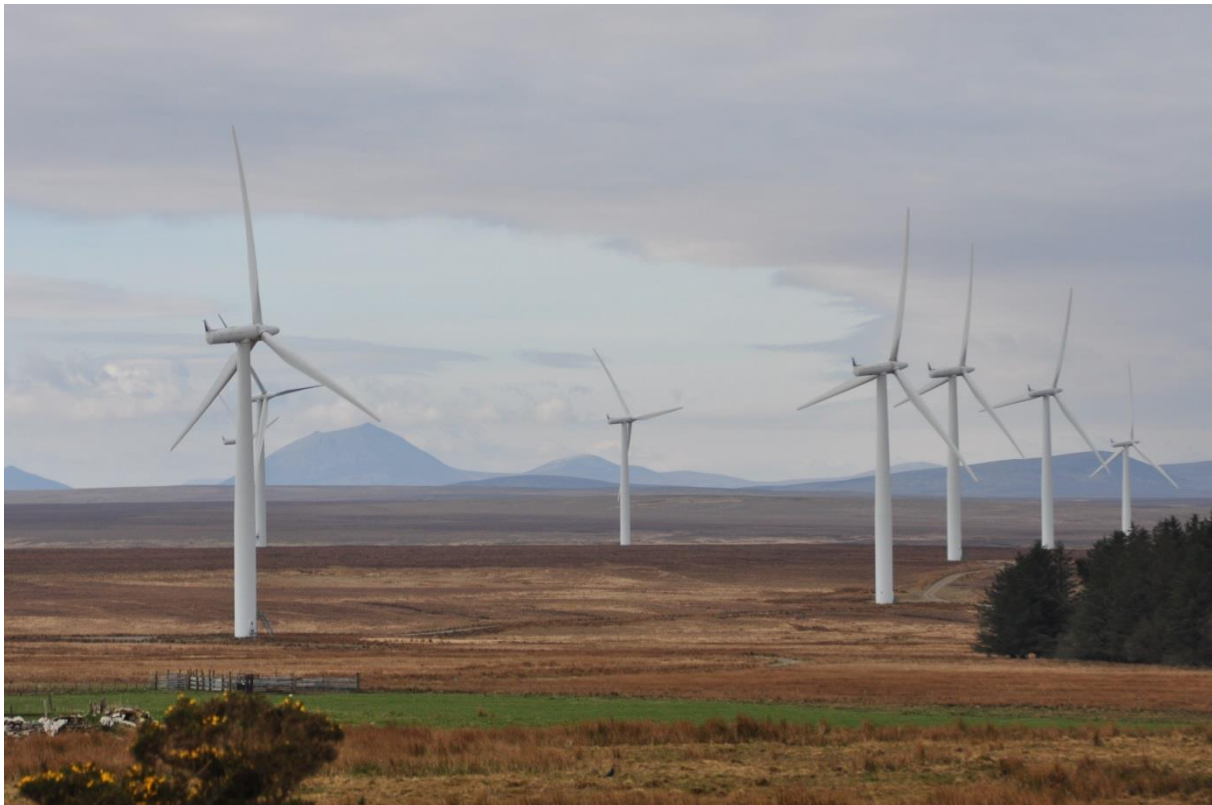
Wind turbines in the Flow Country, Scotland. Photo: Hans Joosten.
