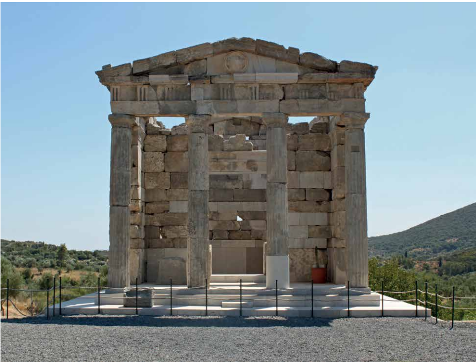
Figure 3. The restored heroon, view from north (photo author).
