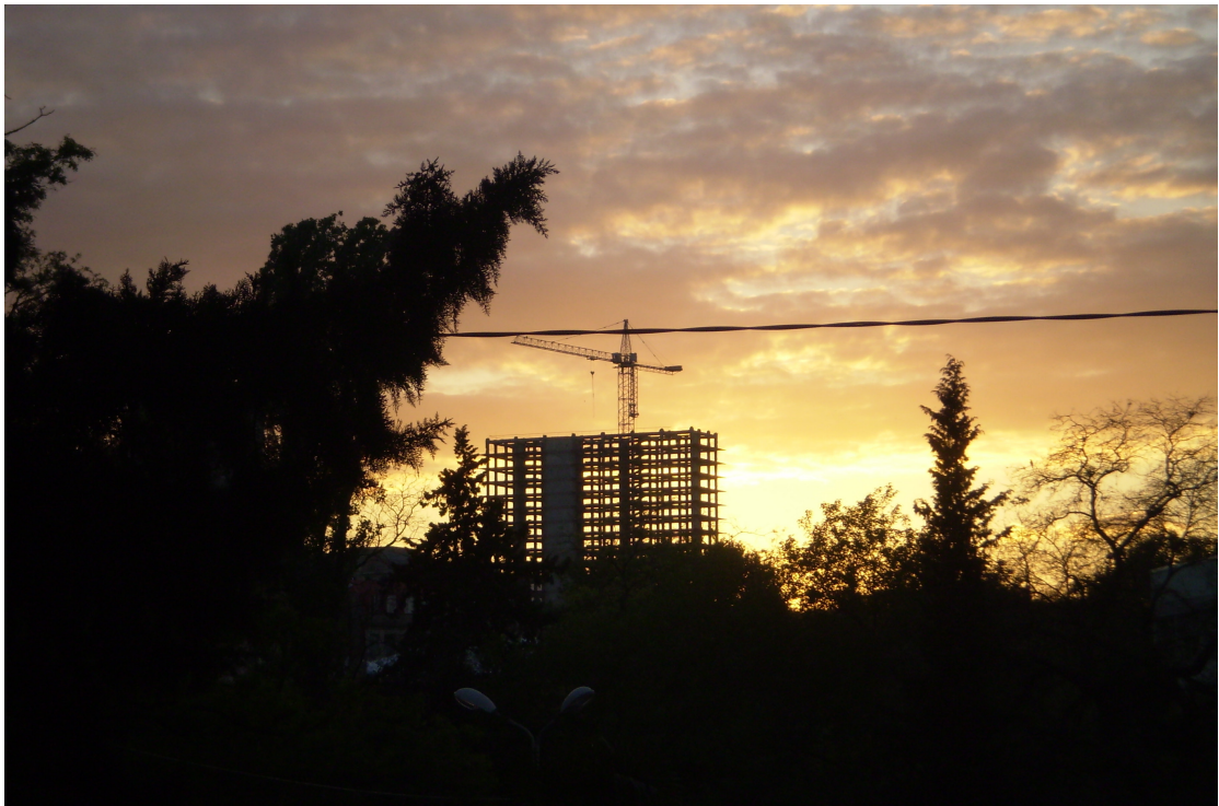
Photo 6: complete renovation of the former IDP-hotel Iveria
