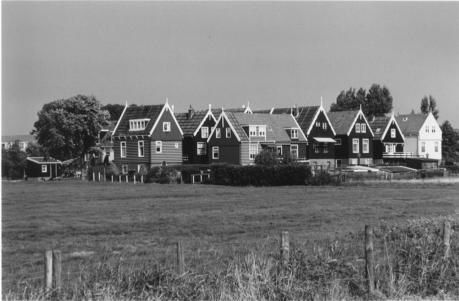
Figure 3: Marken with houses from wood in regional colours
