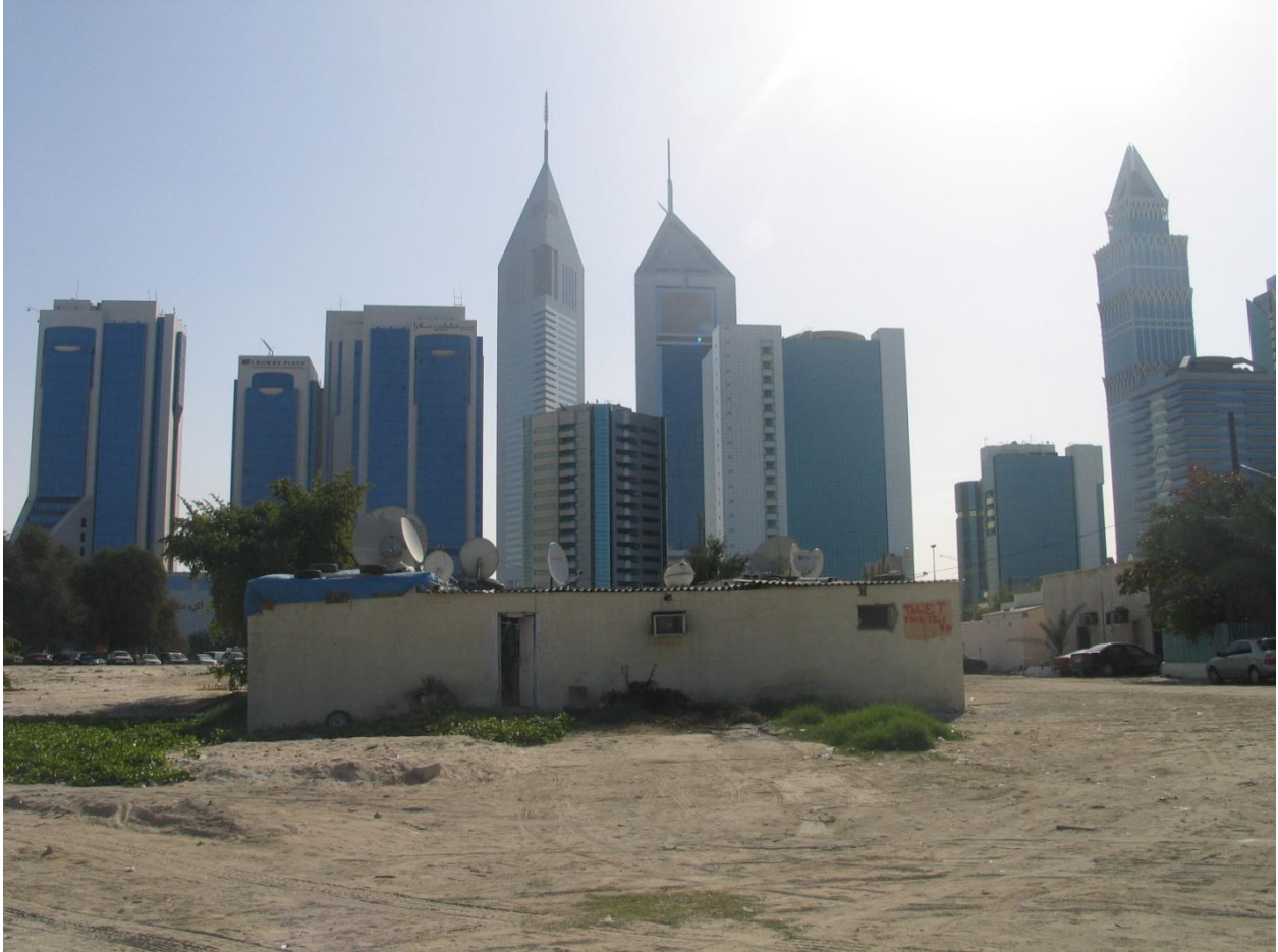
Figure A: An old house that accommodates tens of workers and stands few hundred feet away from the new downtown area. Houses in Al-Satwa are identical in terms of design and construction system. These houses are predominately built of concrete blocks and designed to accommodate all the spaces (including bedrooms, living rooms, and kitchen) around a central courtyard. These houses were not designed by specialists, but by handful of contractors who gained experience in the field. In most cases those builders were called “Oustaz,” an Arabic term of instructor or mentor.
