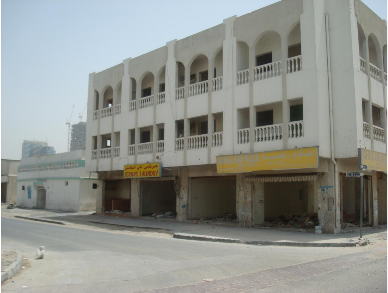
Figure A: A vacant structure waiting its turn to be demolished
