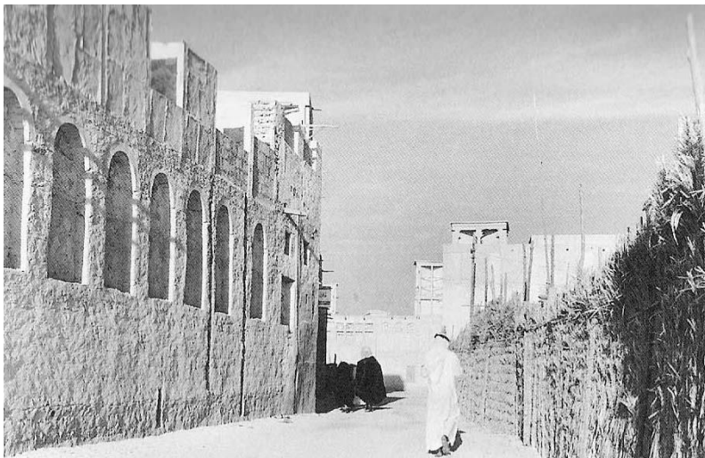
Figure B: A typical pathway and housing typologies. The level of windows in most common cases were above pedestrians' eye level (Facey & Grant, 1996)
