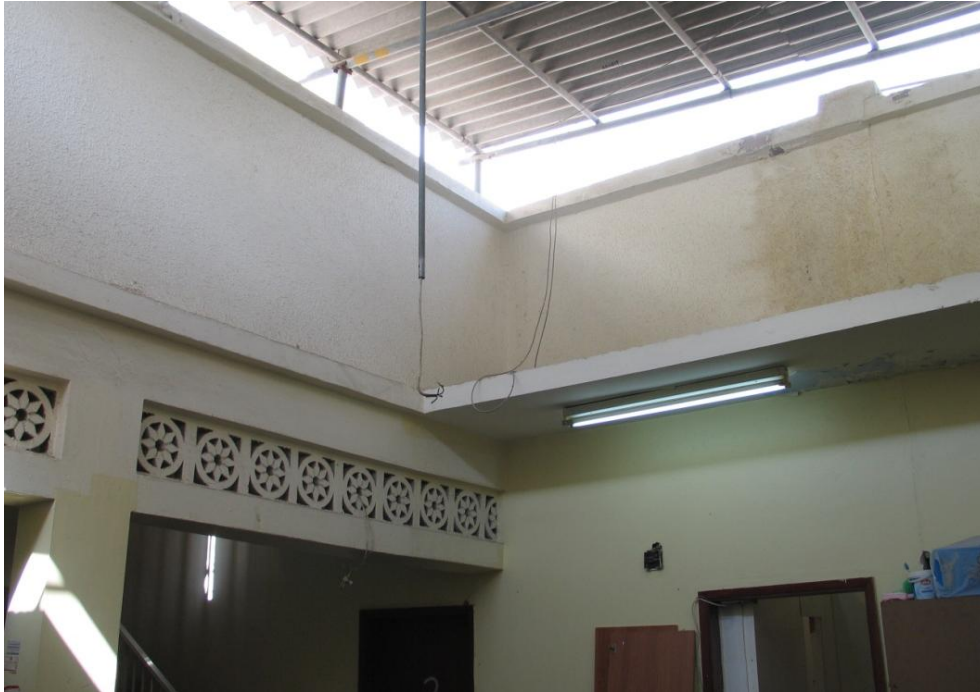
Figure A: A courtyard covered by asbestos to protect the indoor from summer heat and dust. The shading structure is not directly attached to the walls. A little room is left for diffuse lighting and ventilation. In winter, people remove few panels or even the entire panels for the purpose of providing adequate ventilation and direct sunlight.
