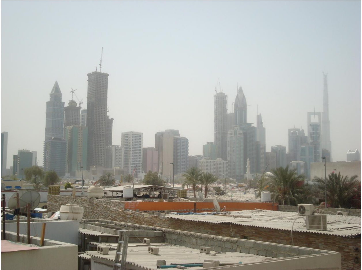
Figure A: Cranes and signs of demolition work in the middle of this shot. What remained in the area is the mix-use corridor known as Al-Satwa busy and dynamic commercial strip and couple of blocks south of the retail corridor. These two blocks that predominantly include low-rise developments with its courtyard typologies are shown in the foreground.
