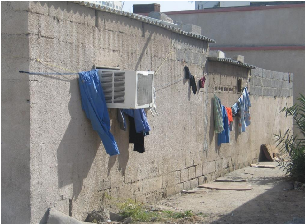
Figure B: Laborers' laundry hanging on walls.
