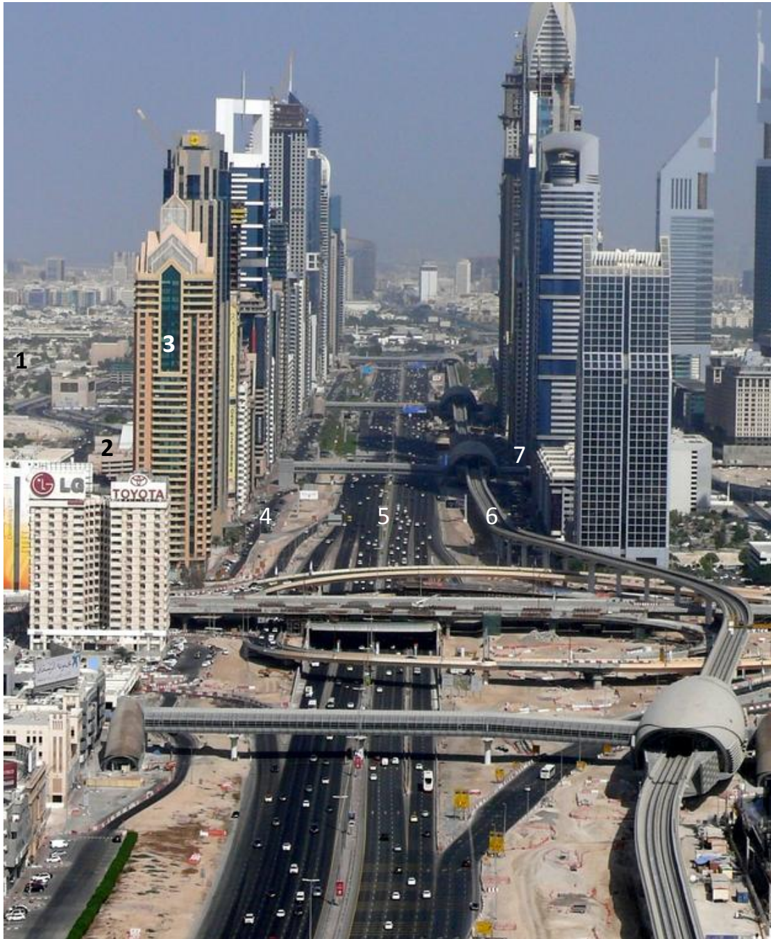
Figure A: From left to right: (1) Subsidized local neighborhoods designed in the early 70s, have deteriorated and are part vacant due to the influx of the working class. In the mid-90s many local families moved to bigger and newer subsidized neighborhoods, leaving the area for the working class; (2) Parking garages, serving the high-rises; (3) Mixed-use high-rise buildings; (4) two lanes of service roads, on-street parking, and a stretch of landscape; (5) A Multi-lane highway; (6) Dubai Metro (The red line that moves along the highway); and (7) Service lanes and high-rises (Skyscrapercity.com)
