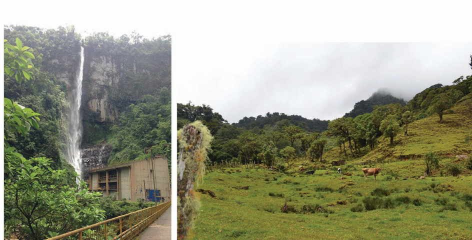
c. Toro III hydroelectric project
