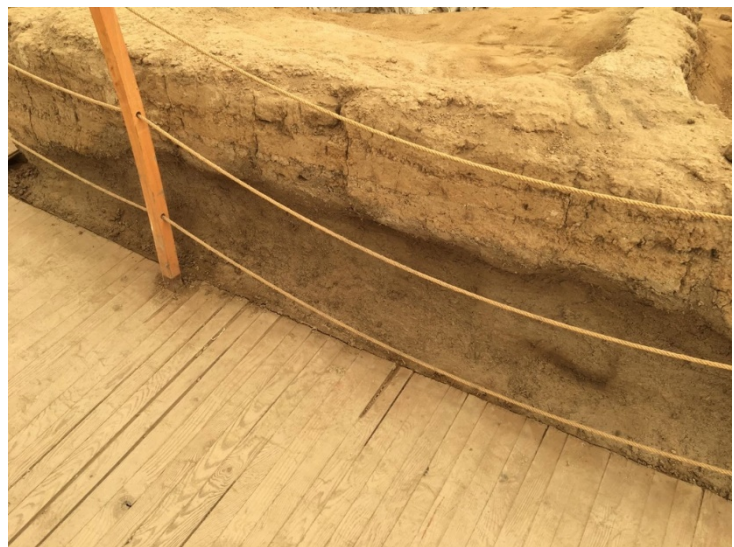
Figure 32: Wall repair on Building 64, undercutting support along the base of the wall. The area is first lined with geotextile, then layers of sieved earth mixed with perlite and chaff are applied to mitigate further erosion.
