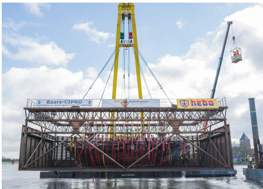
Figure 2. Lifting the IJsselcog, 10 February 2016 (ADC).
