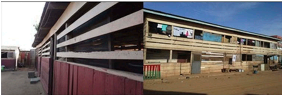
Figure 1. Left: the pilot project (wooden structure); right: transitional housing. Source: Field survey, 2014.
