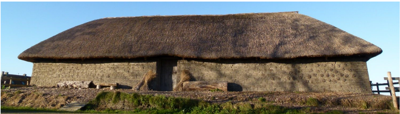
Fig. 6 Experimental reconstruction of an early-medieval turf house on a turf platform in Firdgum. Photo D. Postma.
