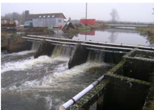
Figure 2: Weir at fish farm. Houtings are unable to progress past the fish ladder on right side of the construction.
