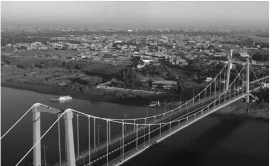
Figure 6: Bridge connecting Tuti Island to Khartoum. Source: Ministry of Information, Republic of Sudan. Khartoum. www.mininfo.gov.S.D , 2014.
